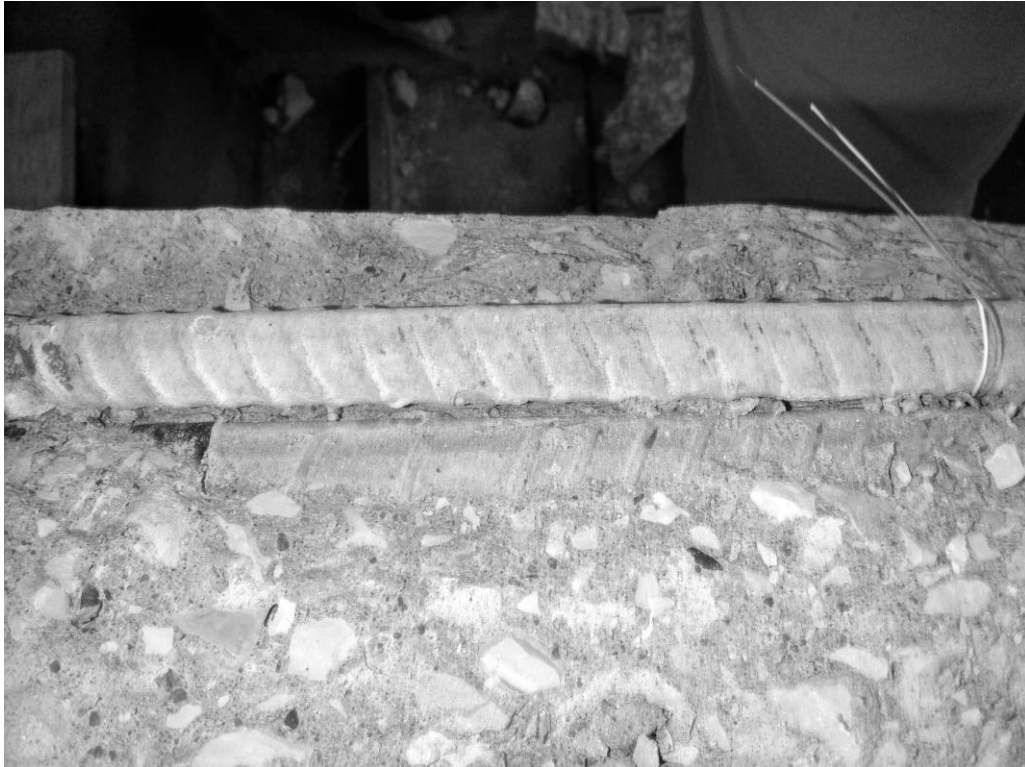
Figure 3.3 Crack pattern in constant moment region of series I
