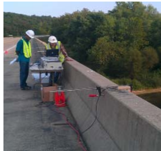
(b) Over Bridge Deck
