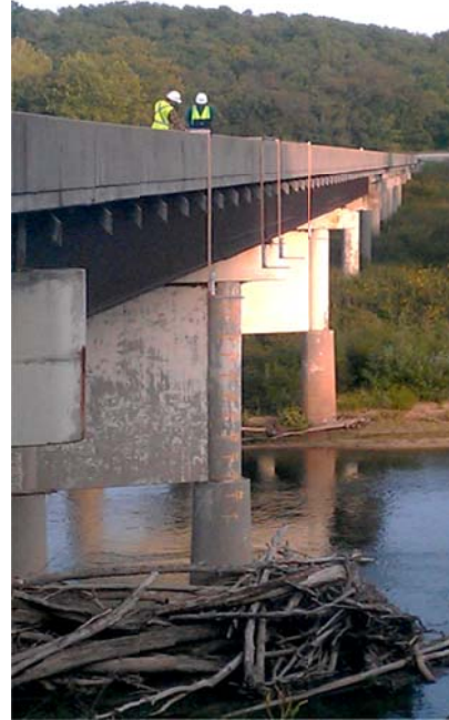
(b) Four Antenna Holders Hung on Bridge Rail
