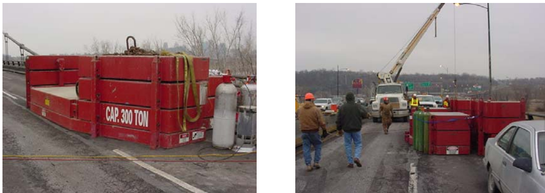
Figure 7.1 Dead Load Ballast Used During Deck Repositioning
