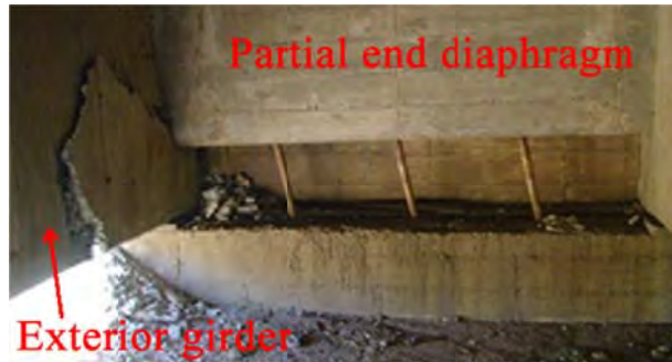
Fig. 3.15 San Nicholas bridge with partial diaphragms.
