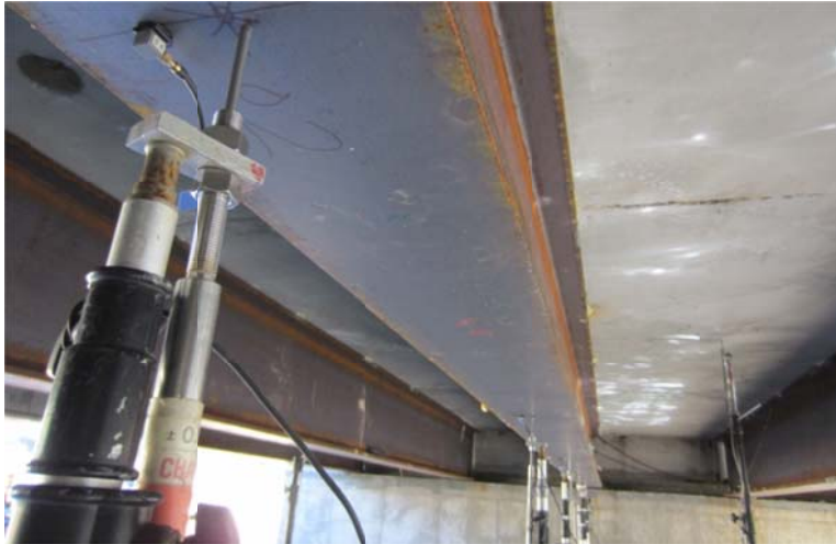
(a) Steel-girder span (7 accelerometers)
