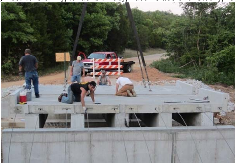
(b) Feeding post-tensioning tendons through deck slabs over concrete girders
