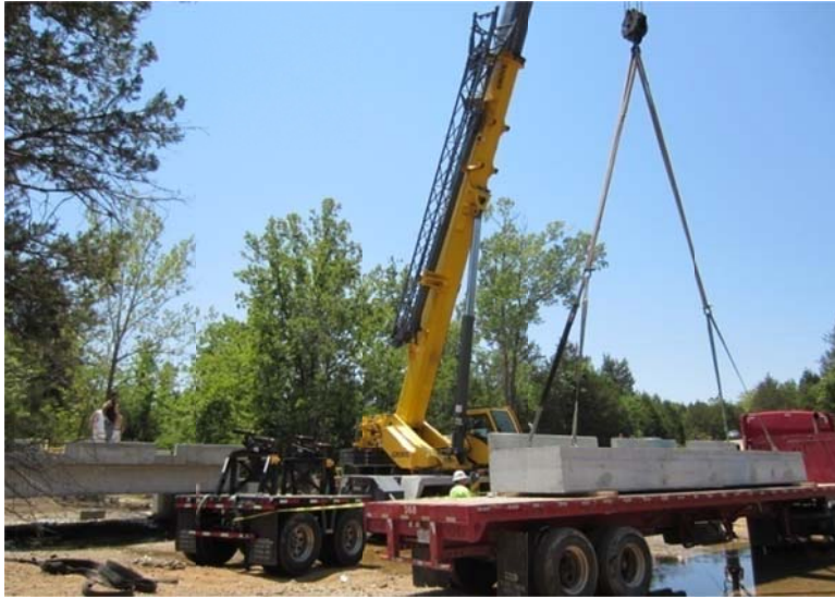
(a) Lifting one box girder
