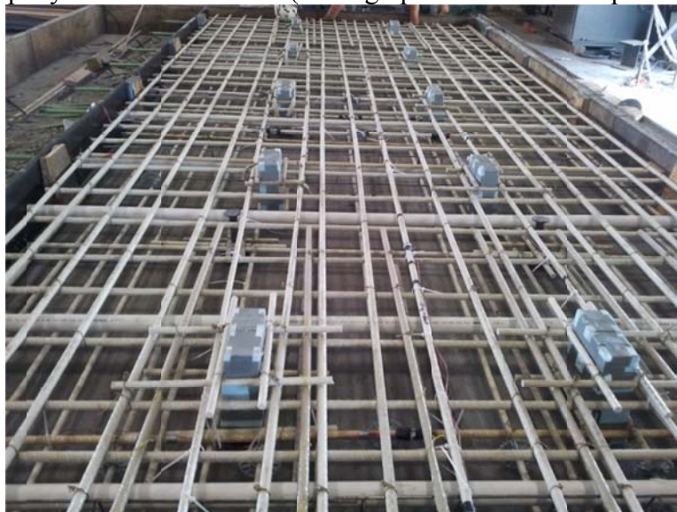
(c) All reinforcement, embedded foams and embedded PVC pipes for post-tensioning
