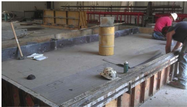
Figure 5.3: Steel formwork for concrete deck slab at the precast plant
