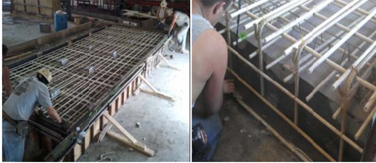
Figure 5.5: Integral construction of bridge curb with deck slab (upside down casting)
