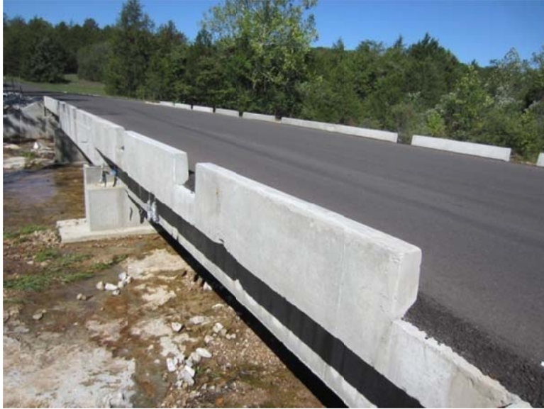
(a) Finished bridge with 3-in. asphalt wearing overlay
