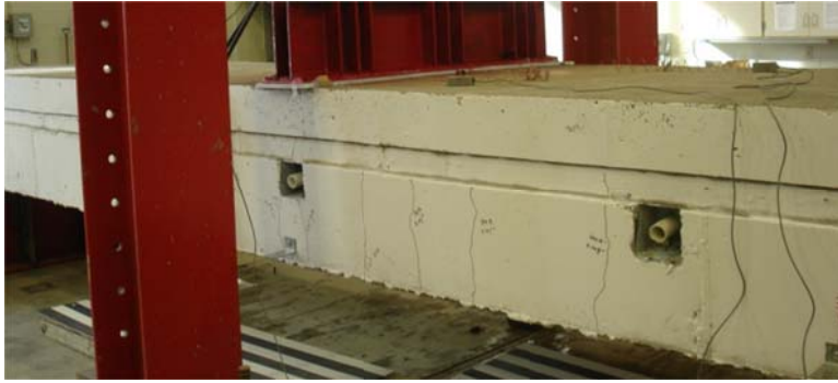
(a) Initial flexural cracks
