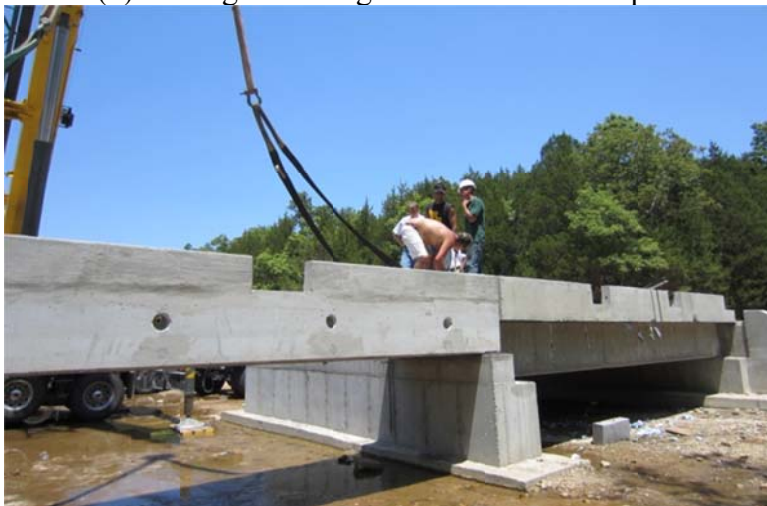
(c) Finishing of one box girder placement
