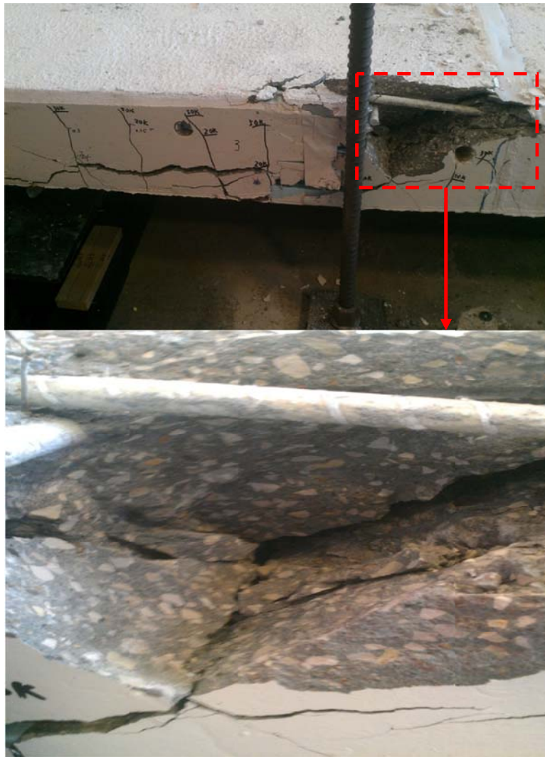
Figure 7.20: GFRP bar condition at shear failure
