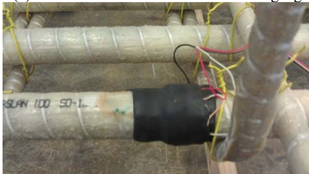
(g) Cover gauges and joints with additional rubber tape
