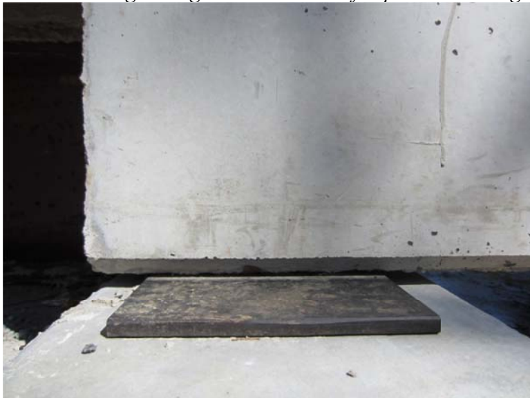
Figure 5.16: Bridge girders seated on a rubber pad
