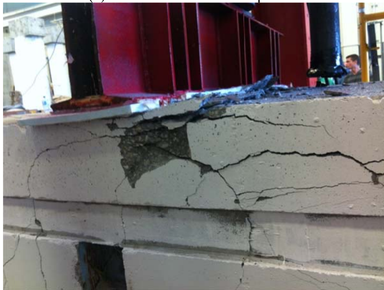
(b) Concrete crushing and horizontal splitting cracks
