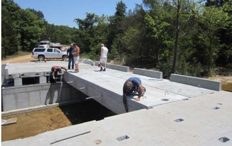
Figure 5.15: Pulling through CFRP tendons for post-tensioning
