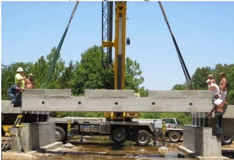
(b) Placing one box girder in the middle span
