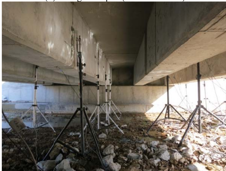
(c) Concrete-girder span (20 DC-LVDTs)
