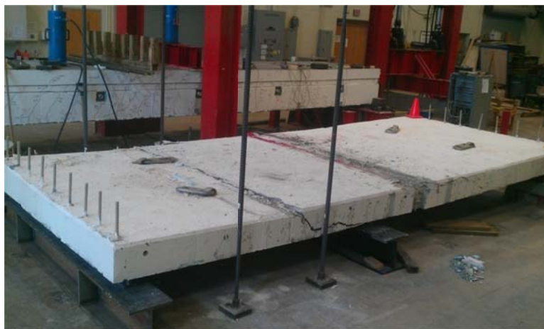
Figure 7.21: Overview of the collapsed slab after two load cases
