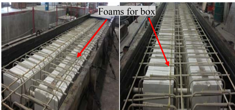
Figure 5.7: Formwork for concrete box girder
