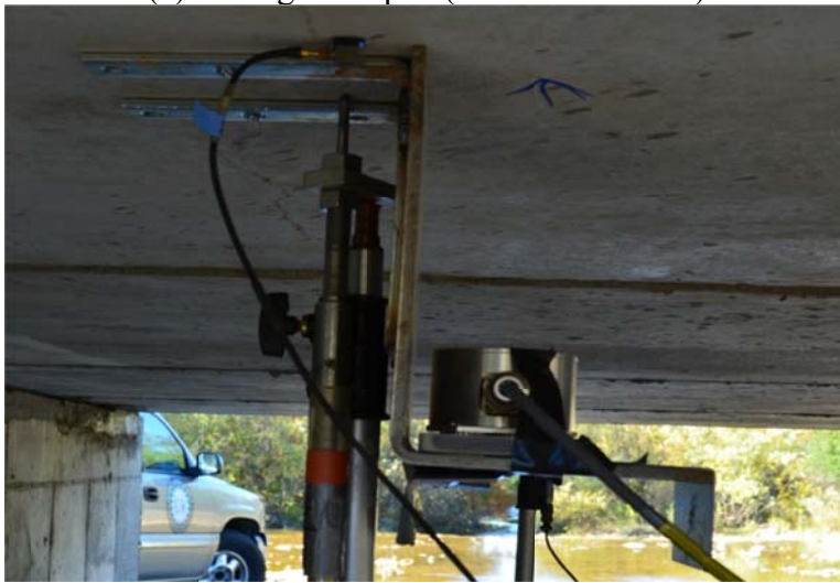
(b) Box girder span (7 accelerometers)
