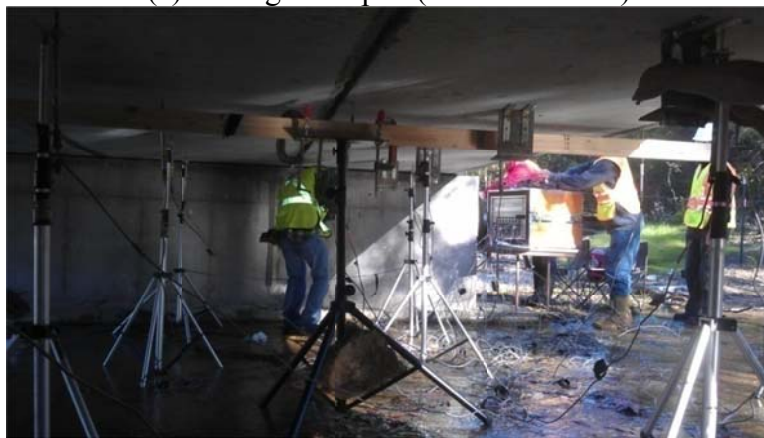
(b) Box-girder span (20 DC-LVDTs)
