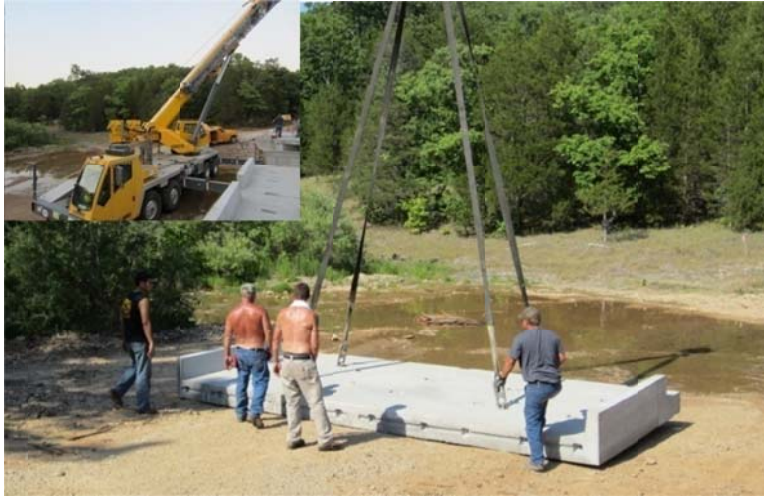
(a) Uplifting one deck slab by a crane
