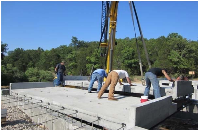
(a) Post-tensioning tendons through deck slabs over steel girders
