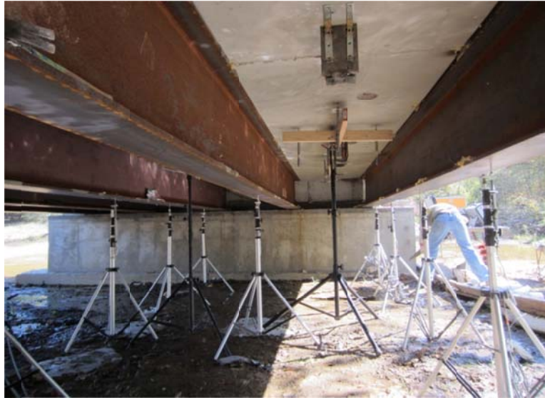
(a) Steel-girder span (20 DC-LVDTs)
