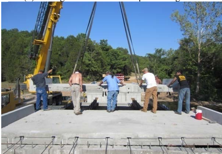
(c) Placing second concrete deck slab
