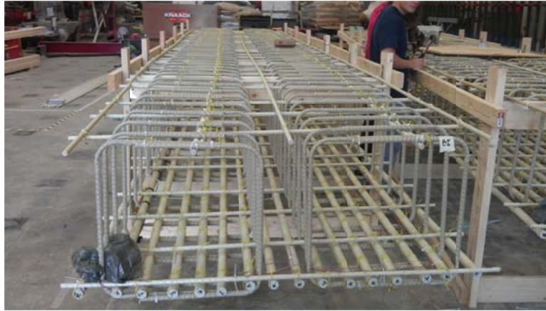
(a) Box girder cage with installed strain gauges
