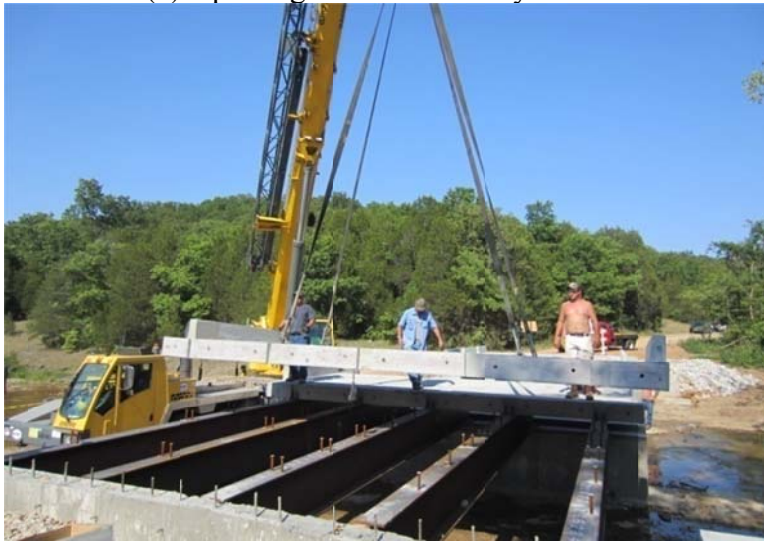
(b) Placing one deck slab on top of steel girders
