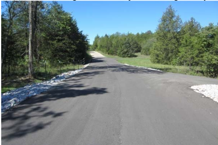
(b) East approach roadway
