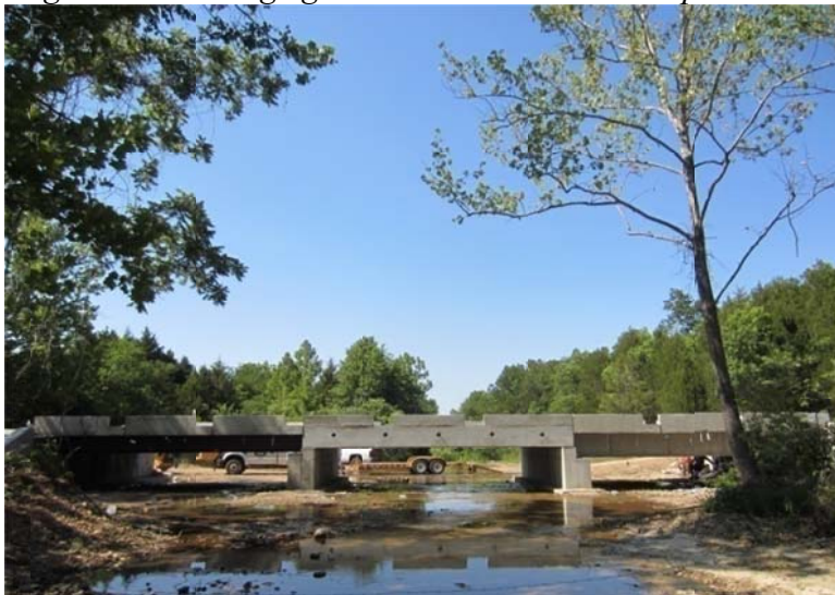
Figure 5.17: The newly erected three-span bridge
