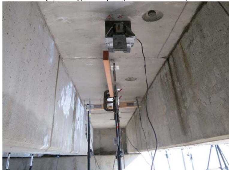
(c) Concrete-girder span (6 inclinometers)
