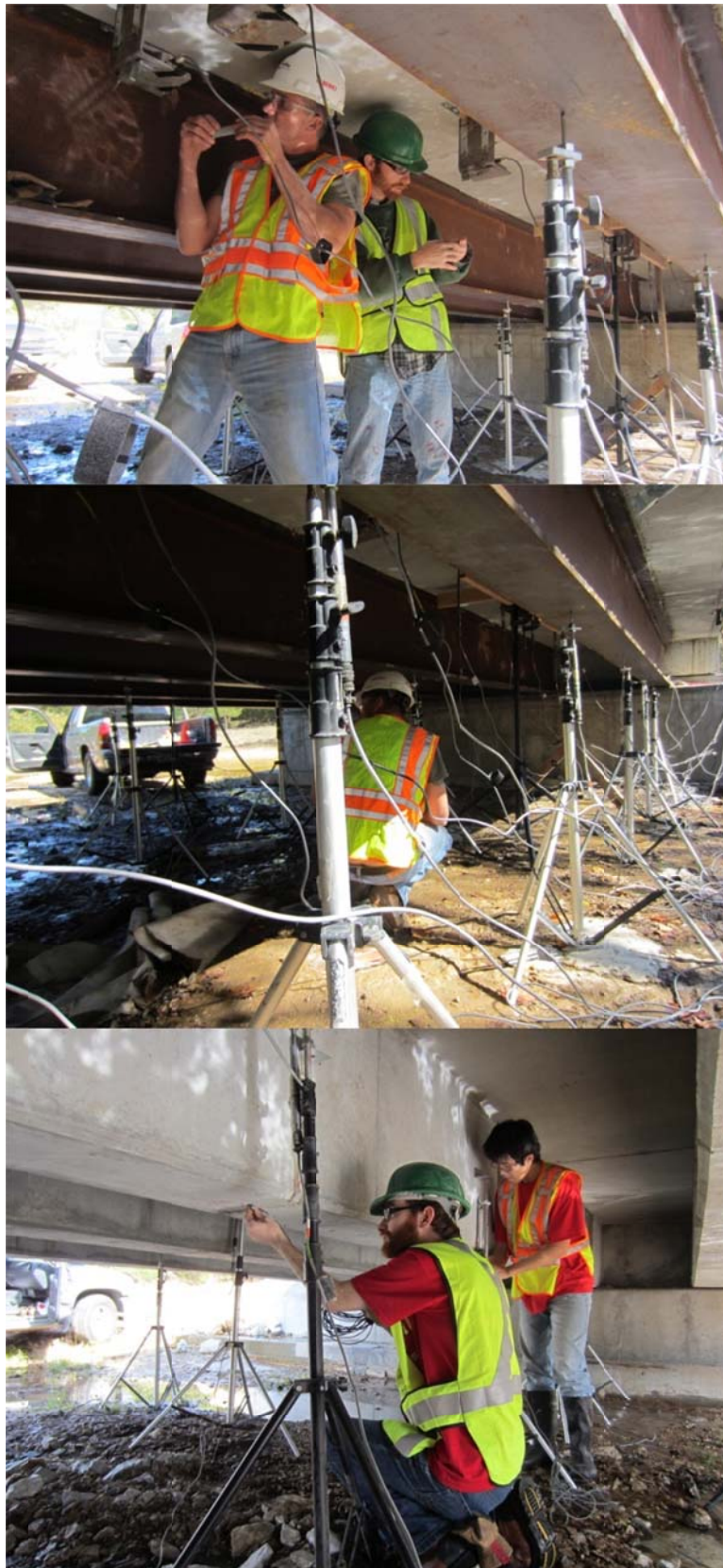
Figure 6.18: Installation process of representative sensors
