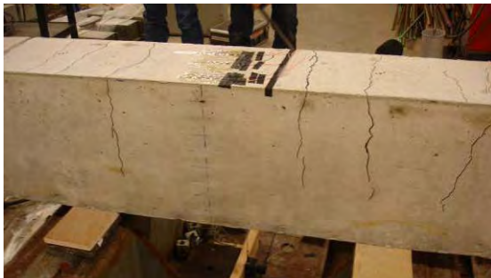
(b) Initial cracks
