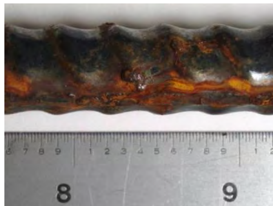
(b) “Significant” signs of corrosion
