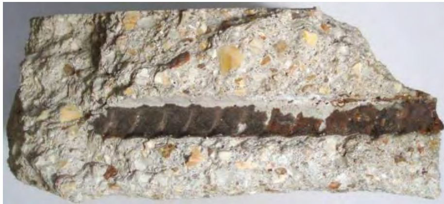
Figure 6.46 Red rust stayed on the concrete surface of a 50/50 enamel specimen.
