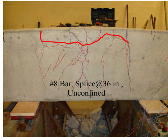
(f) Split failure of B-8-2 with steel yielding
