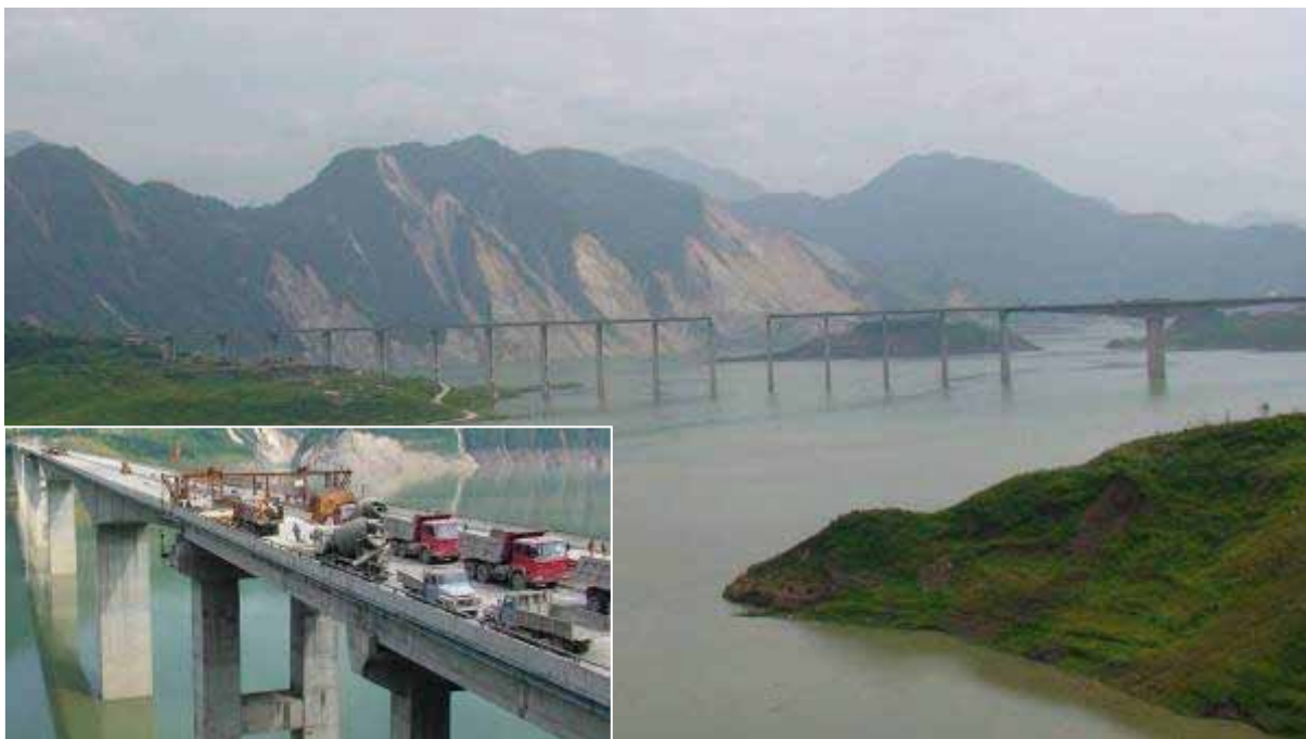
Figure 54. Photo. Overview of Miaozhiping Bridge.
