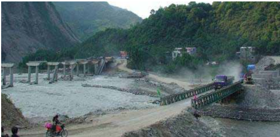
Figure 49. Photo. Overview of Temporary Bridge Construction.
