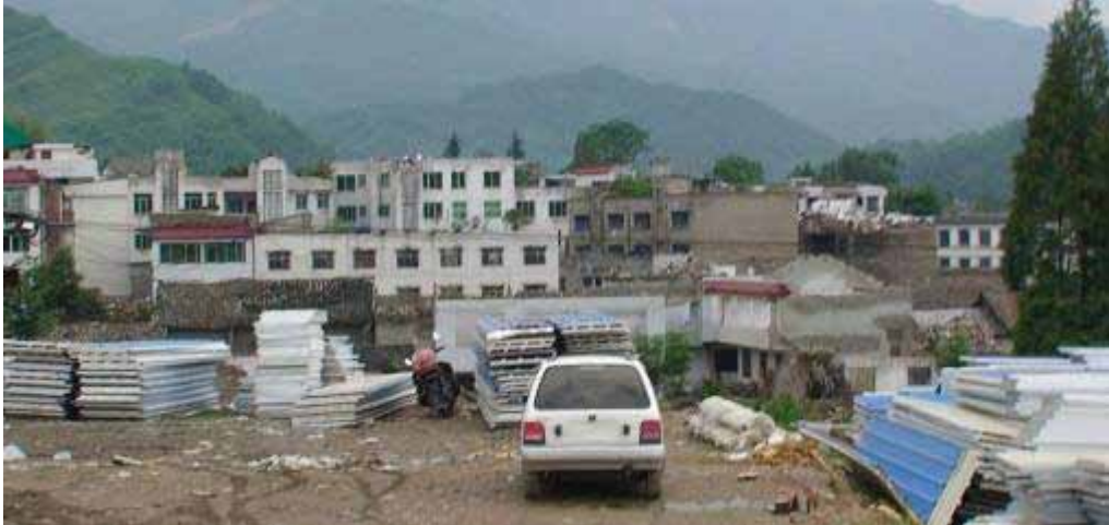
Figure 11. Photo. Building Damage Near Zhima Bridge.
