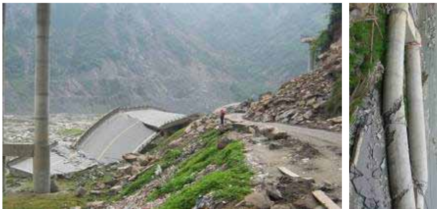
Figure 68. Photo. Column Shear Failure and Section 5 Collapse at Bent 15.
