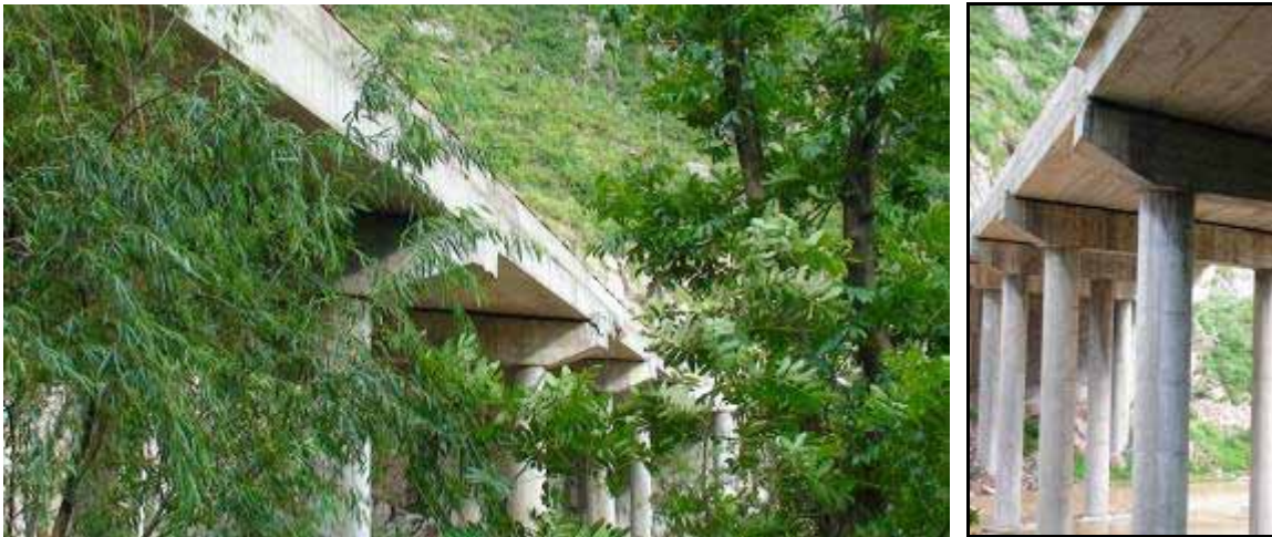
Figure 30. Photo. Overview of Baimayan Bridge.
