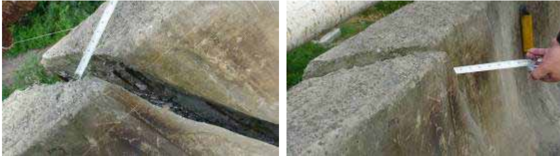
Figure 32. Photo. Measurement of Expansion Joint Offset.
