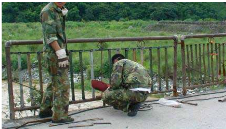
Figure 10. Photo. Welding on Bridge Railings.
