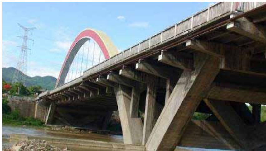
Figure 25. Photo. Part of the Anzhou Bridge.
