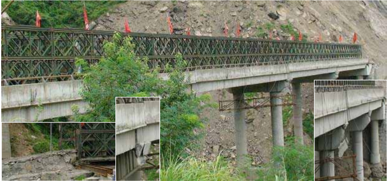
Figure 73. Photo. Bailey Bridge Over the Existing, Damaged Bridge.
