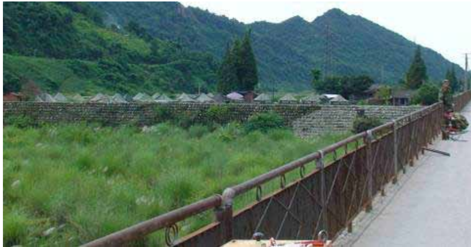
Figure 12. Photo. Tent Area Near the Bridge.
