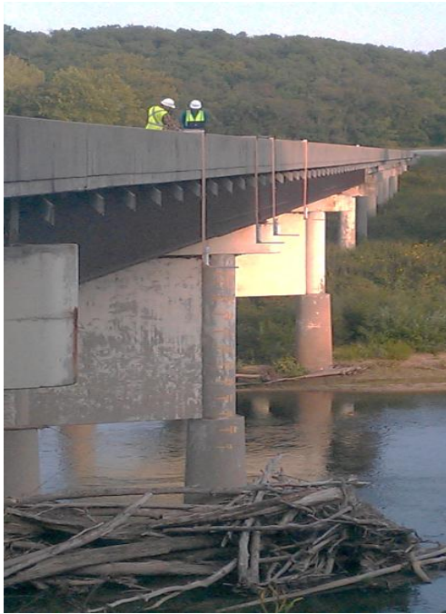
Figure 20. US 63 road bridge
