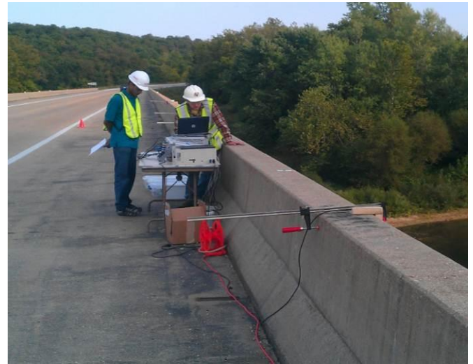
Figure 23. US 63 road bridge – bridge deck base-station location
