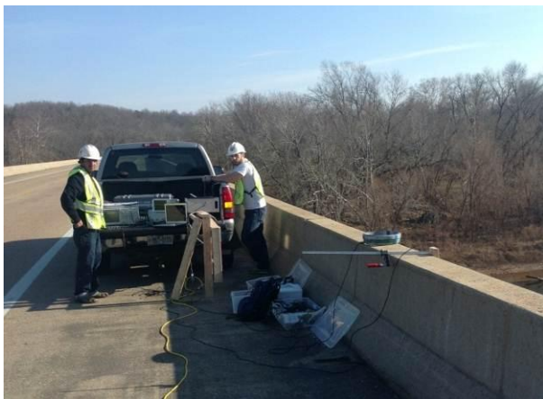
Figure 26. US 63 road bridge – Bridge deck location
