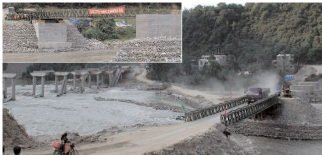
FIGURE 5 Construction of a temporary bridge.
