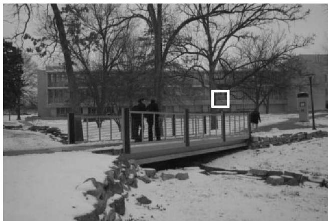
Fig. 1. Smart Composite Bridge at the UMR. The location of the dedicated Web camera is indicated on the building in the background.
