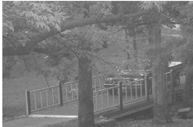
Fig. 2. Frame acquired from dedicated Web camera of the SCB. The traffic-monitoring exercise uses the right parking light of the truck as a marker for tracking.
