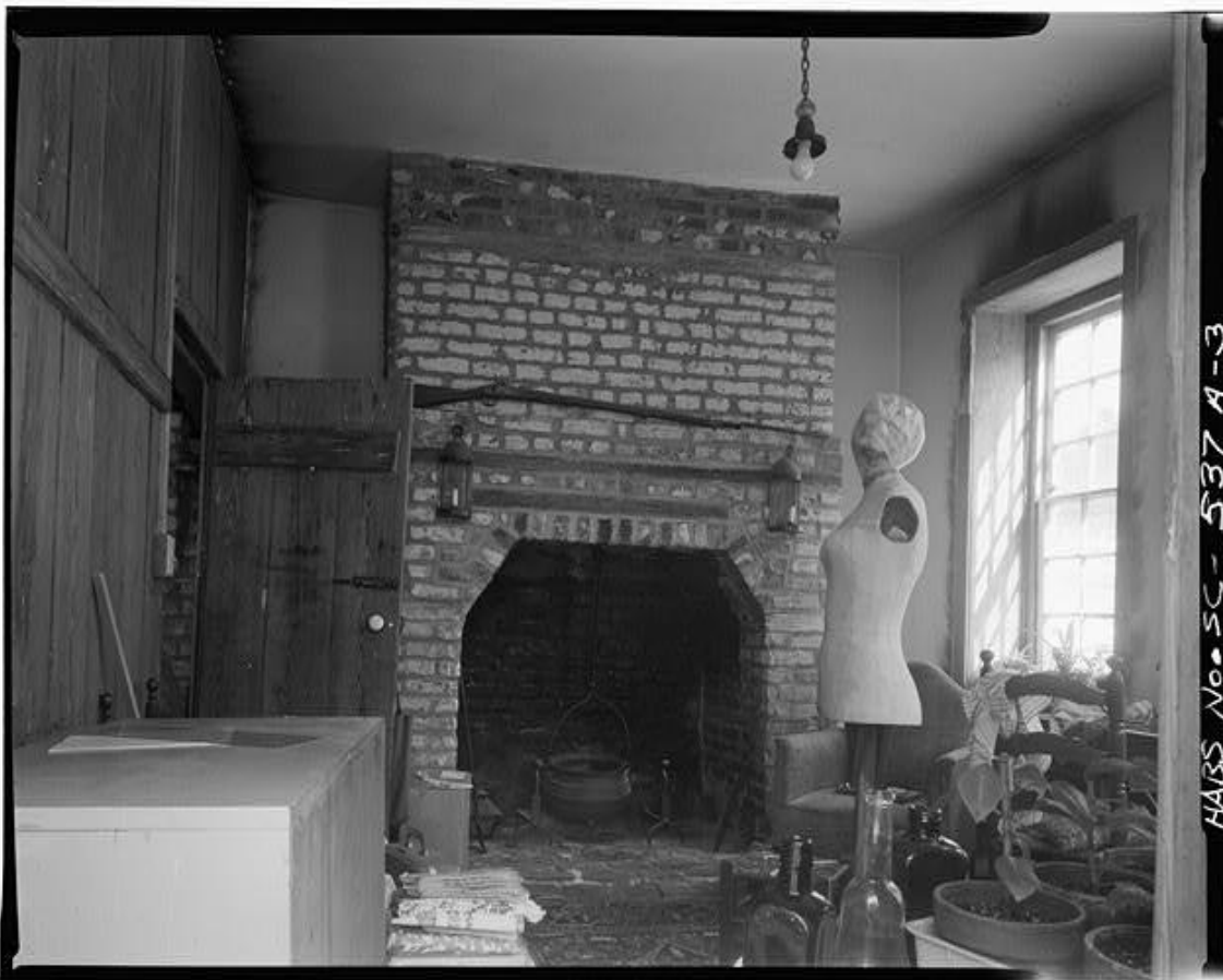
Figure 10. Photograph of Dr. Samuel Crane Kitchen Building, 4 Orange Street, Charleston, Charleston, SC. (HABS SC,10-CHAR,333A-3, 1978)
