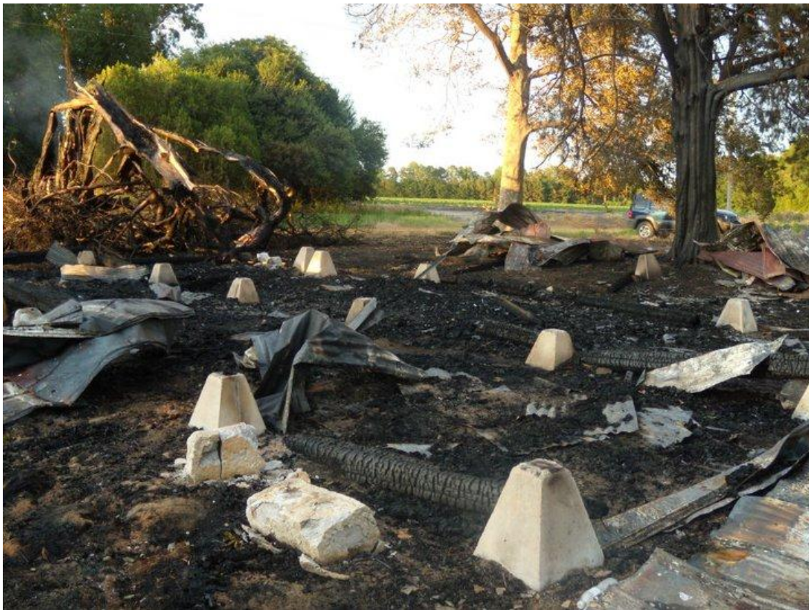
Figure 47. Photograph showing an Early 20 th Century out building constructed of beam over pilings support. Burnt 7/22/11 in Register, GA. View #1
