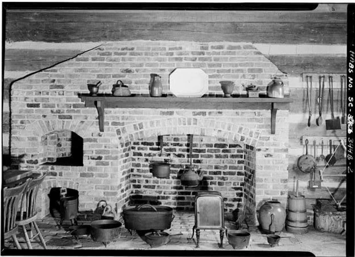
Figure 42. Fort Hill, Kitchen, Clemson University Campus, Pickens South Carolina. Taken by Jack E. Boucher 1960. Shows the interior view of fireplace and brick oven. Shows common display and storage of kitchen-wares (HABS SC, 39-CLEM, 1B-2, 1960)
