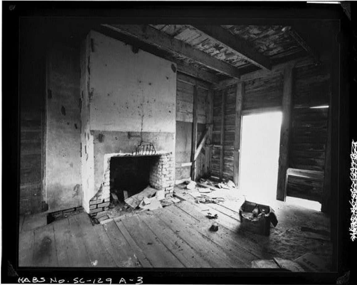
Figure 7. Photograph of Kensington Plantation, Summer Kitchen, U.S. Route 601, Eastover vicinity, Richland, SC. Interior View of Hearth (HABS SC,40-EAST.V,1A-3, 1982)
