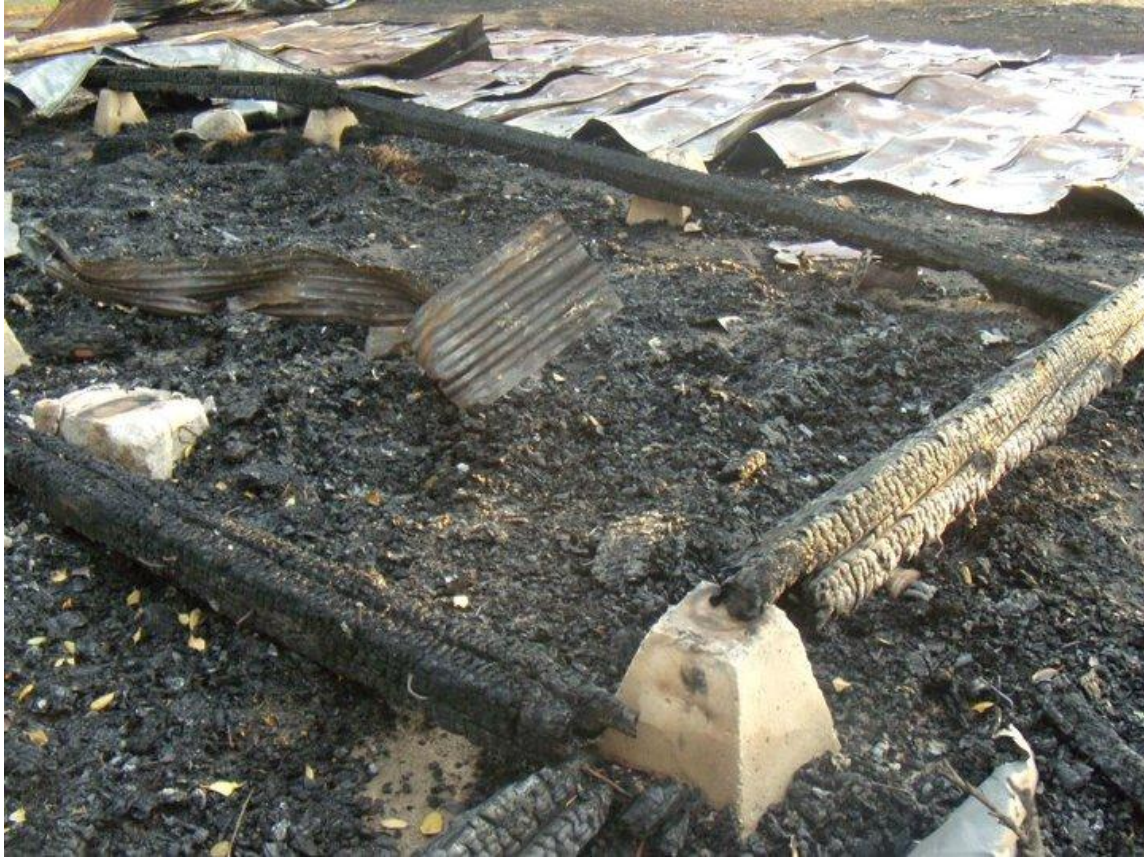
Figure 48. Photograph showing an Early 20 th Century out building constructed of beam over pilings support. Burnt 7/22/11 in Register, GA. View #2
