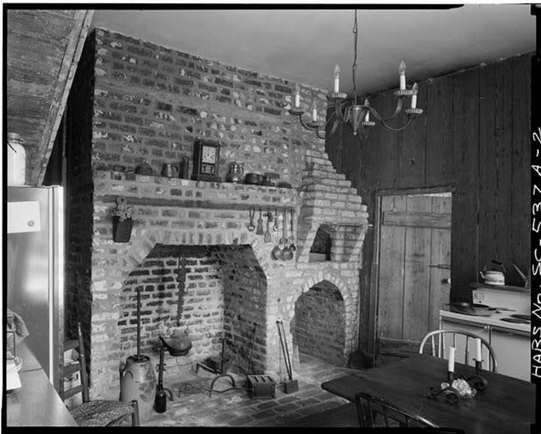
Figure 9. Photograph of Dr. Samuel Crane Kitchen Building, 4 Orange Street, Charleston, Charleston, SC. (HABS SC,10-CHAR,333A-2, 1978)
