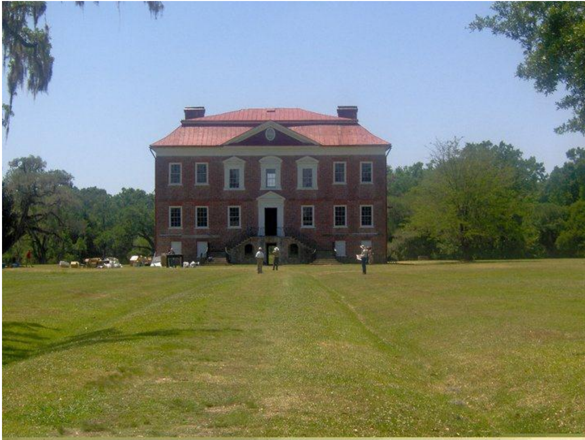
Figure 1. Photograph of Drayton Hall view from the Ashley River, front main entrance of the home
