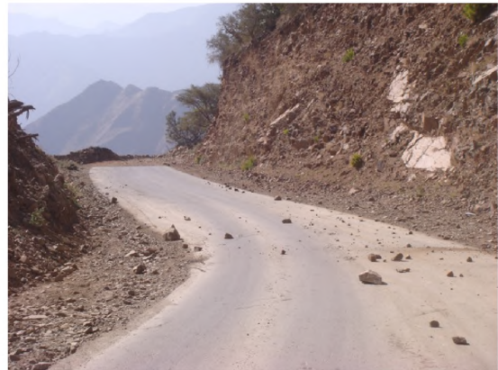
Figure 3. Characteristics of the Raidah escarpment road. (note, one lane with a 3 meter width for each direction)
