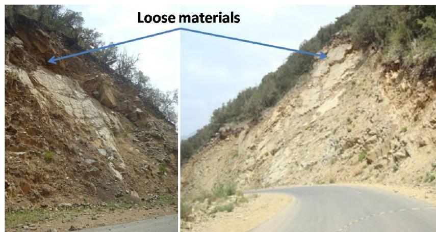
Figure 20. Shows loose materials need to be scaled from some sites
