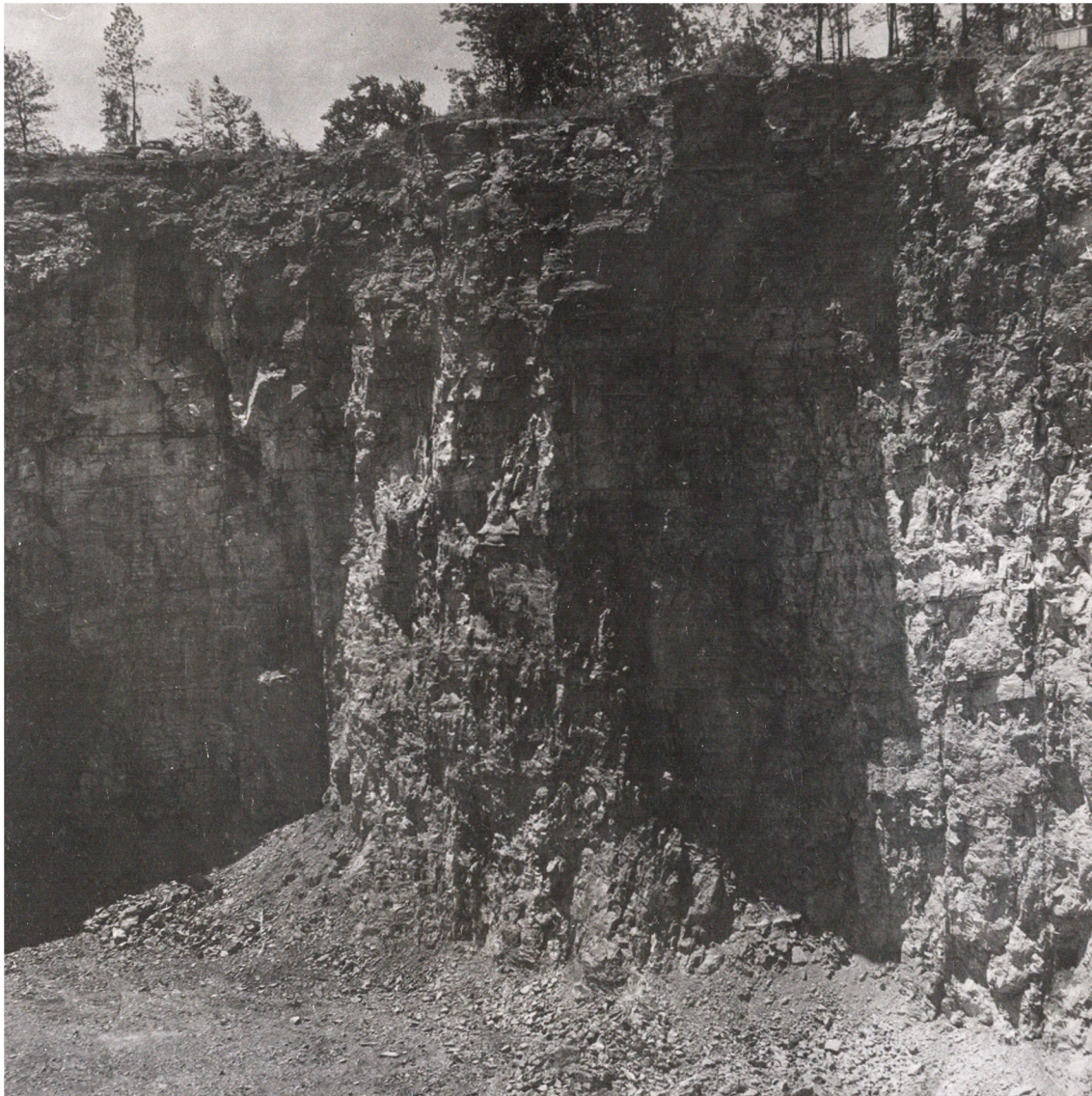
CORNER FRACTURE FORMATION QUARRY FACE BEFORE INITIATION COURTESY OF ATLAS POWDER COMPANY
