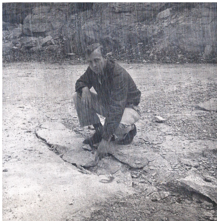
Plate 6. Crater Formed in Horizontal Free Face From Test Number 2.
