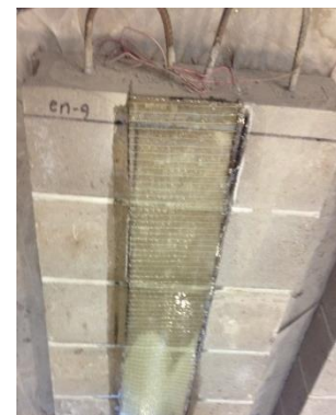
Apply saturated sheet on wall
