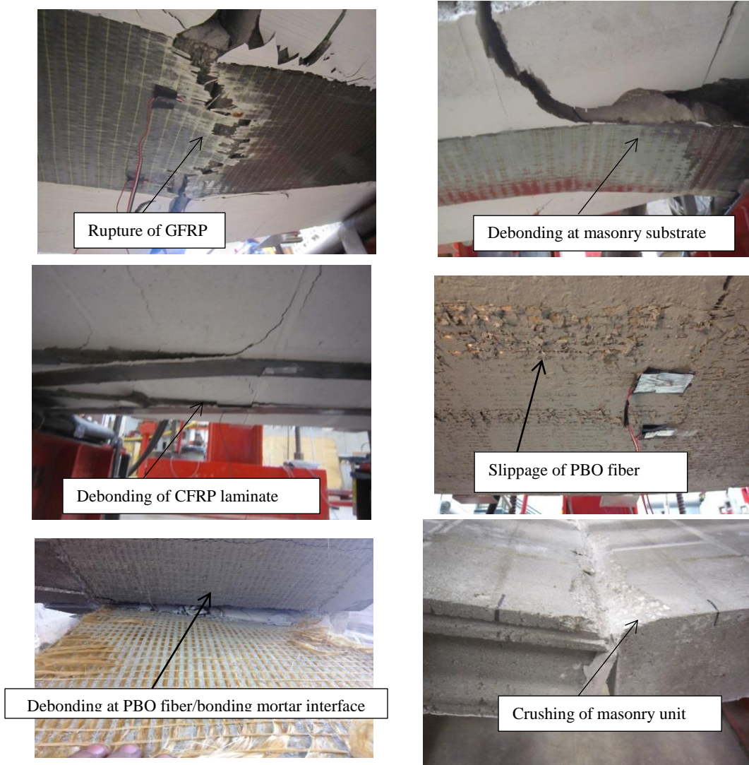
Figure 6. Typical mode of failures
