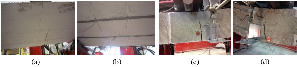
Figure 6. Crack development during load testing (a) block mortar crack, (b) masonry unit cracks, (c) flexural cracks, (d) flexure shear cracks
