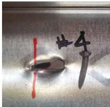
Figure 7: Shear Bearing of 33 mil CFS track (concrete base material)
