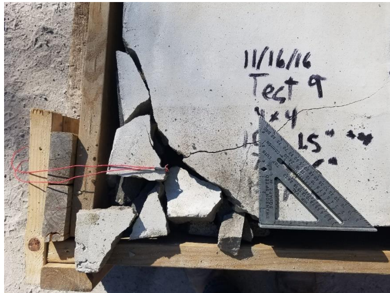
Figure 33 Top Layer Breakage Test 23
