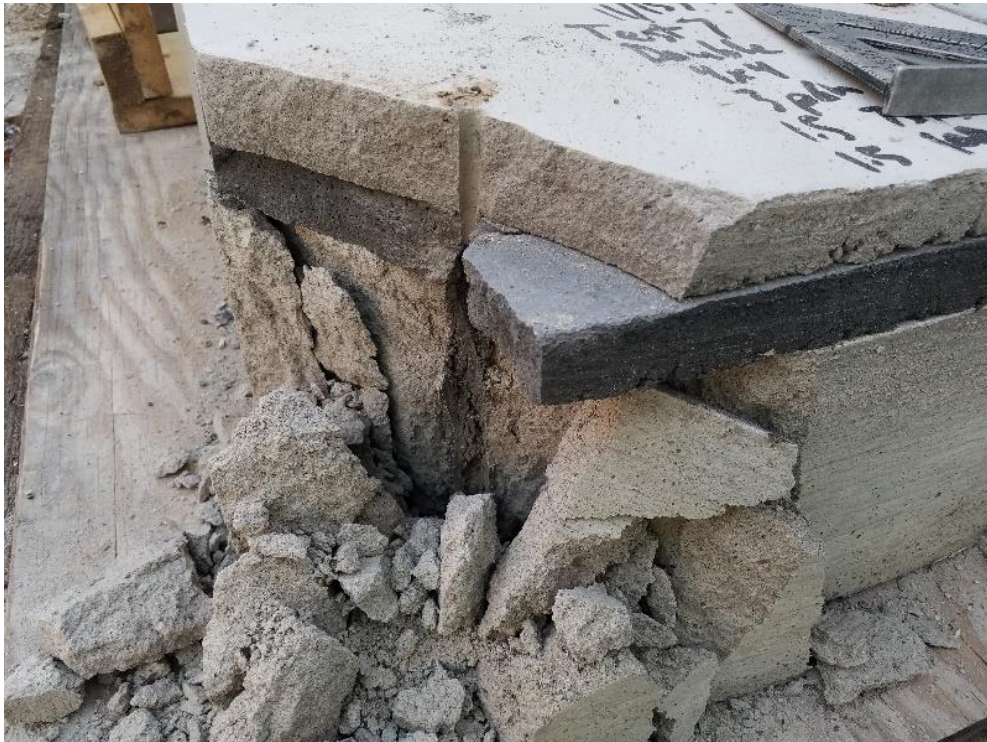
Figure 5.6. 3-Layer Test Block Post-Blast, Test 21 11/15/16
