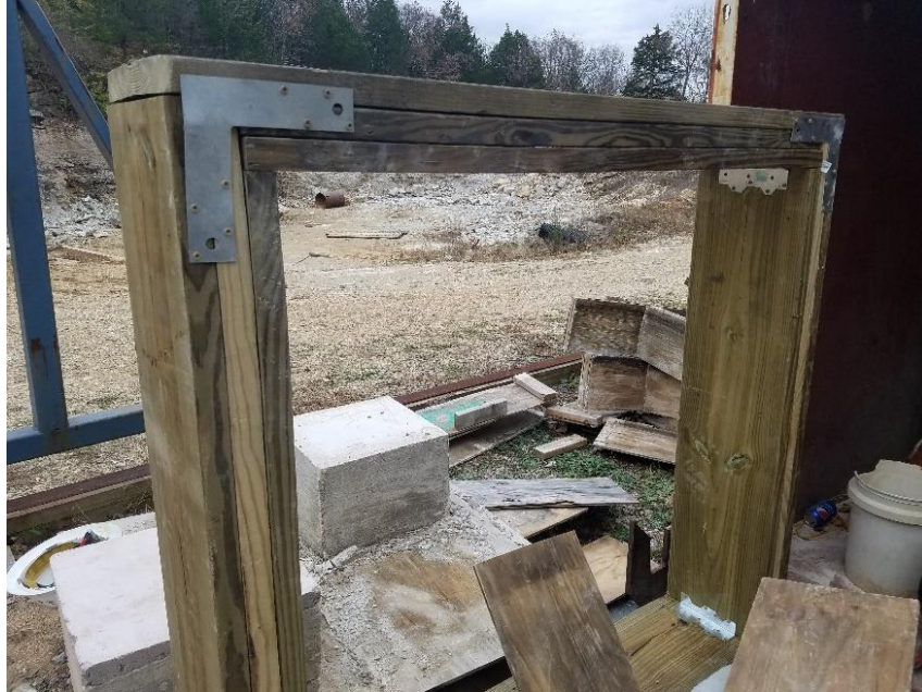
Figure 4.5. Reinforced Crib Construction
