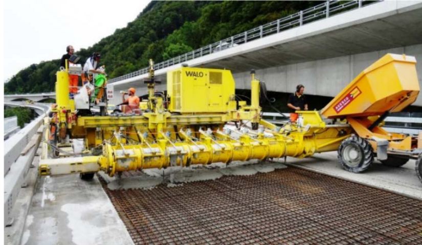
Figure 2-16 Implementation details of UHPC overlay application
