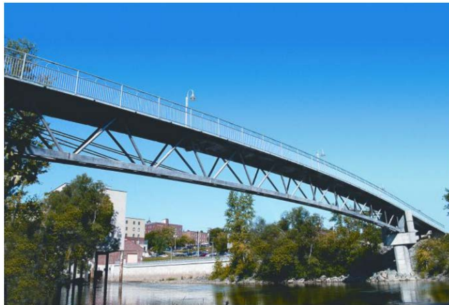
Figure 2-12 Sherbrooke Pedestrian Bridge (Russell and Graybeal, 2013).
