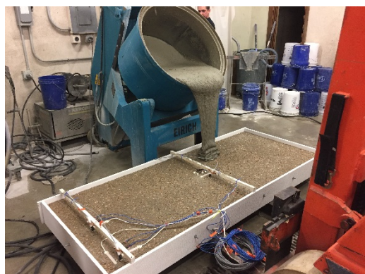
Figure 6-6 Preparation and casting process of UHPC overlay
