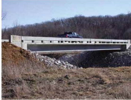
Figure 2-14 Mars Hill Bridge, Wapello County, IA, USA (Russell and Graybeal, 2013)
