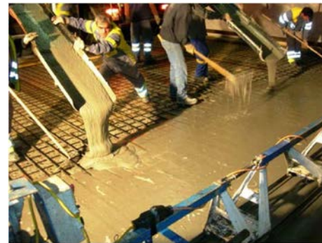
Figure 2-6 Cross section (dimensions in cm) with UHPFRC layer (in grey) and view of UHPFRC casting performed (Bruhwiler and Denarie, 2008)
