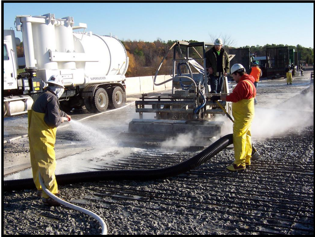
Figure 1.8: Hydro-demolition ( www.flickr.com )
