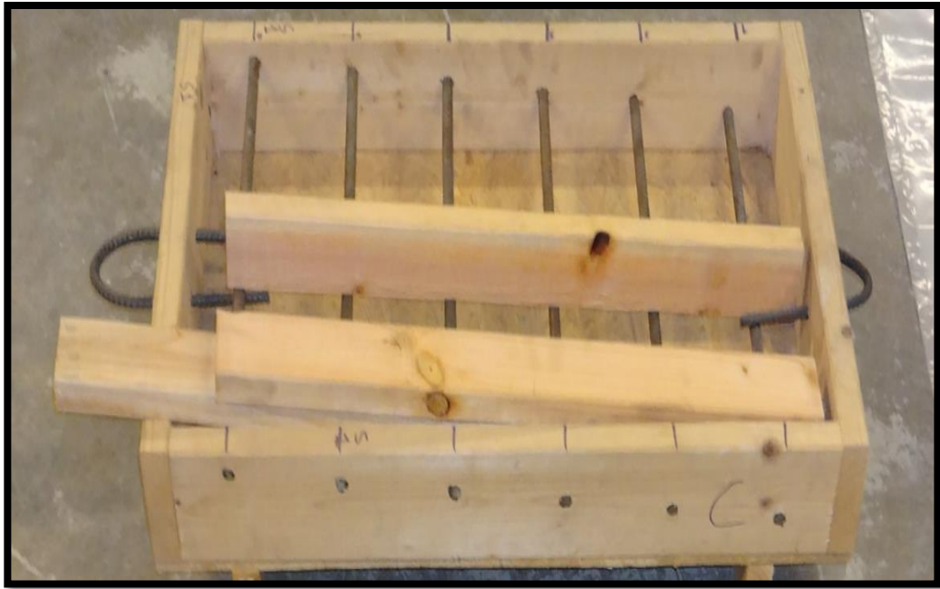
Figure 2.2: Slab-1 before pouring concrete (courtesy Aleksey Khamzin)
