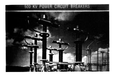
Figure 10. 500 kV Air Blast Circuit Breaker
