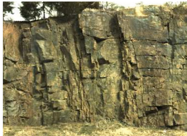
Fig. 11 Rock cut selected for verification study.
