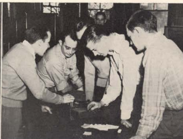
Checking the voltage. Briefing.
