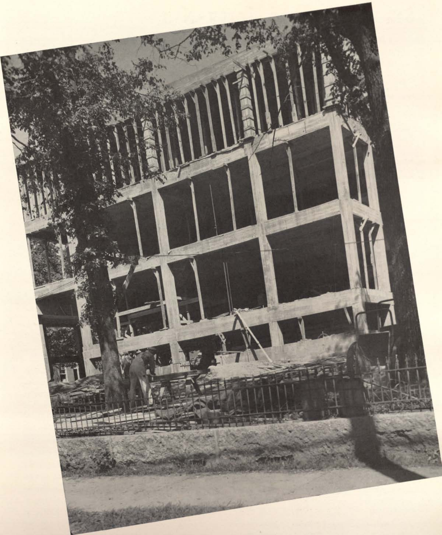
Addition to Chemical Engineering Building - - - September, 1948
