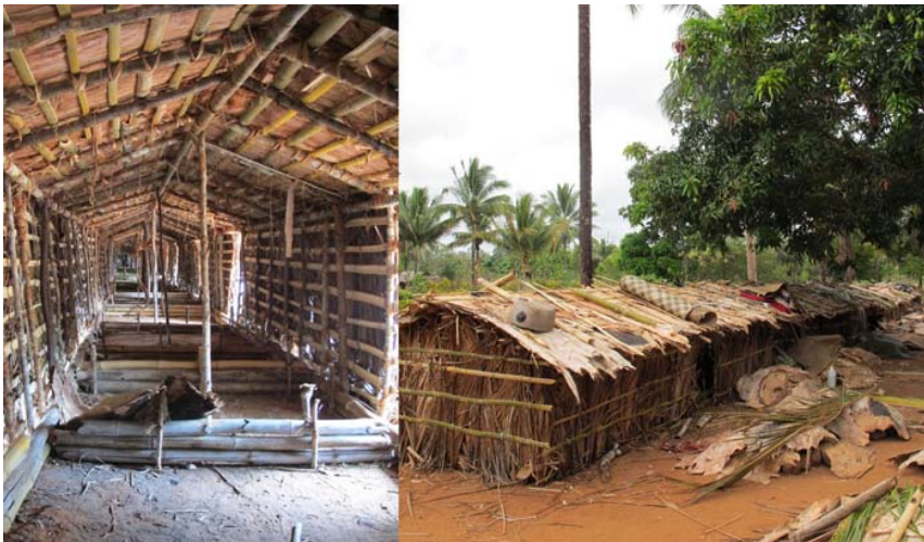
Figure 1.14: Communal yamhouse in Yokwa: inside (left) / outside (right)
