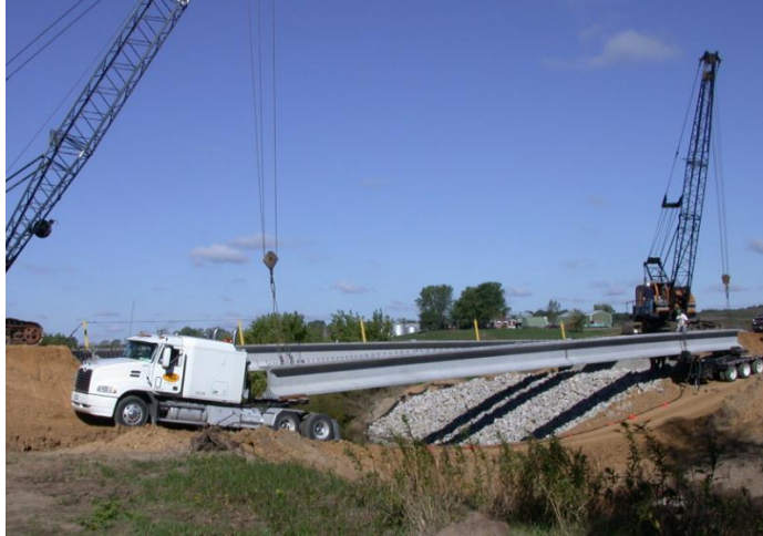
Figure 1.3. Mars Hill Bridge in Wapello Country Iowa, 2006, USA. (Aaleti et al. 2011)
