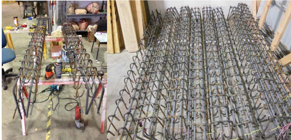
Figure 9-11 Fabrication and instrumentation of reinforcing cages.
