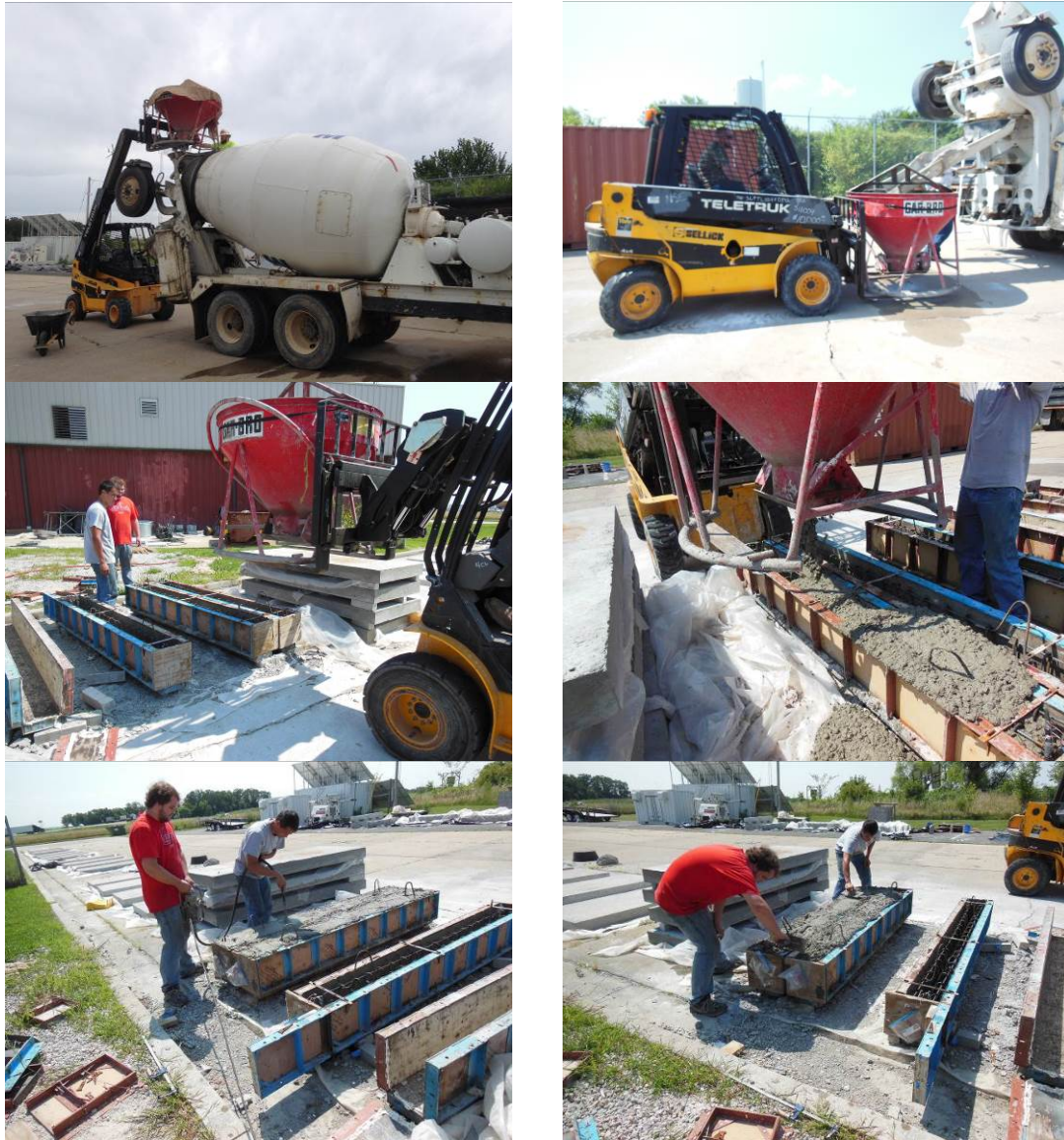
Figure 9-15 Concrete beam construction procedures.
