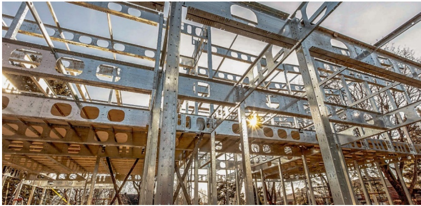
Fig. 1. Perforated light gauge beams (Bone Structure, 2005)
