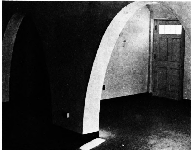
Fig. 8. Individualized archways for custom designed rooms
