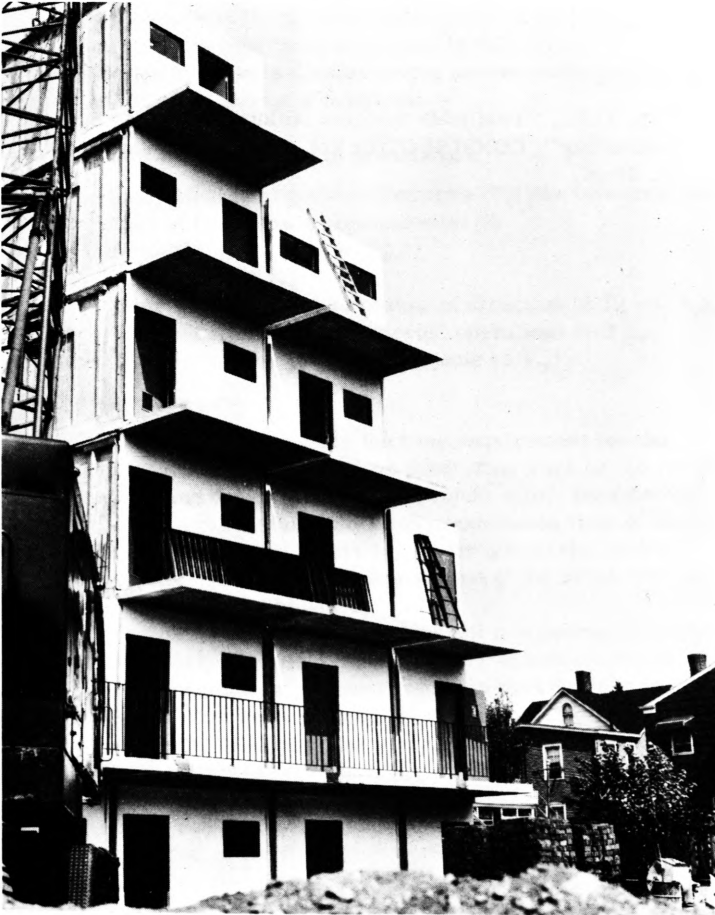
Fig. 7. Field erection of modules
