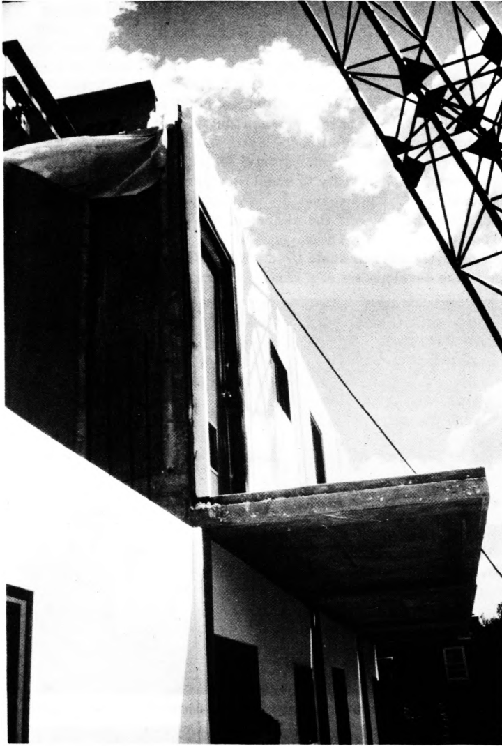
Fig. 10. Construction view of reinforcement for front and back columns
