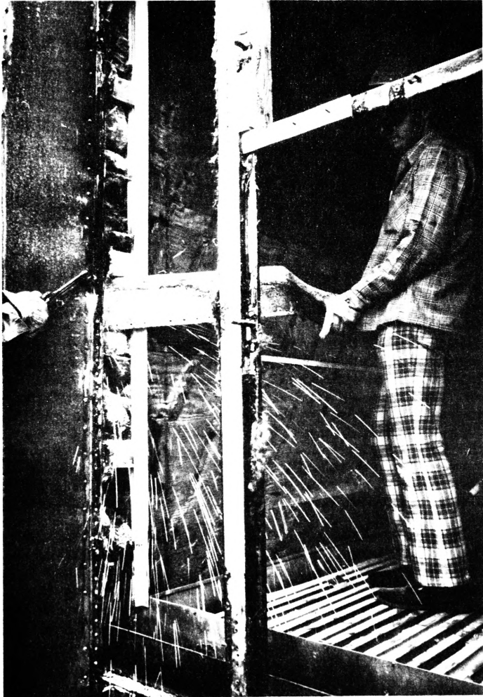
Fig. 5. Cutting Steel Members
