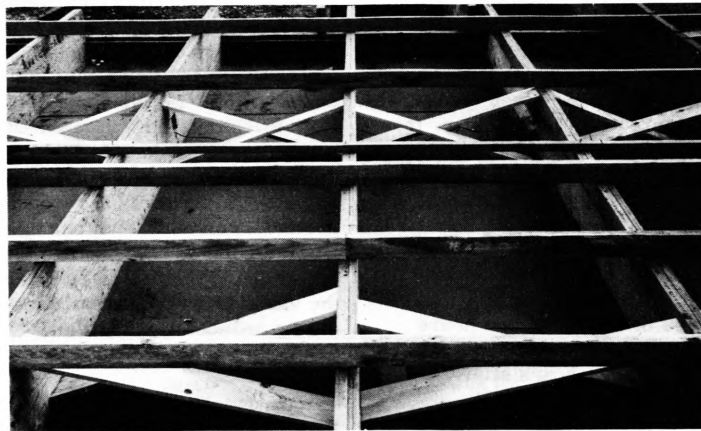
Fig. 4. Floor Plenum Area in Construction
