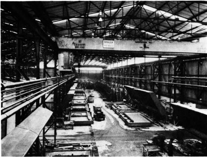
Fig. 7. Permanent Factory for Balency System, Thamesmead, England.
