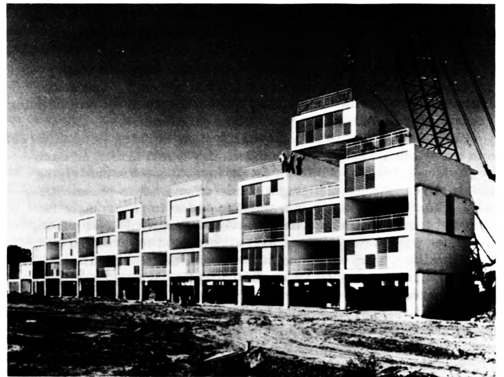
Fig. 5. Shelley Box System, Puerto Rico.
