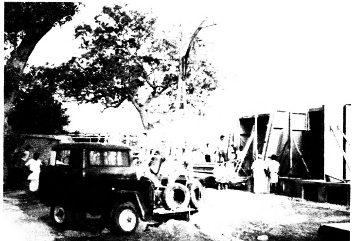
(b) - Hoist assembled on a jeep seen in the front of picture and scooter hoist-in the back of picture. (Sand bags used as counter balance).
