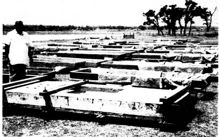
Fig. 5 Example of timberform for wall panels used in North Bengal. In front - freshly cast window wall panel. In the back - panels in curing.
