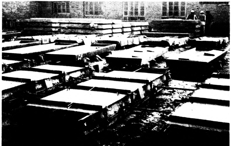
Fig. 6 Example of steel form for casting of UCOPAN panels for roof/floor, used in Nepal.
