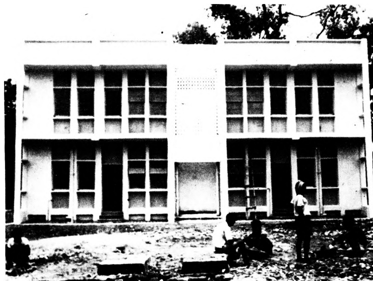
Fig. 25 Illustrations of construction of two-storey apartment house made of standard UCOPAN panels, erected as a prototype in Calcutta.
