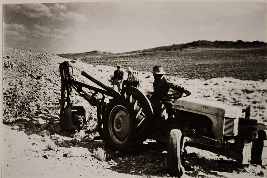
Figure 50. Mica pit (Pegmatite No. 12), Mechanical shoveling of waste rock.
