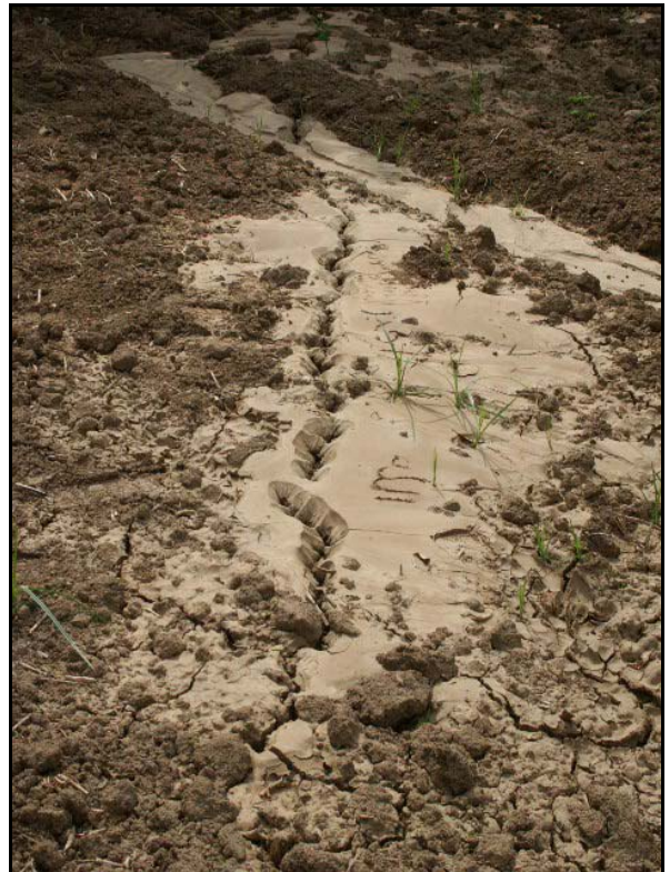
Fig. 16. Liquefaction-induced sand boils and sand flow into an irrigation ditch in Zemmouri
