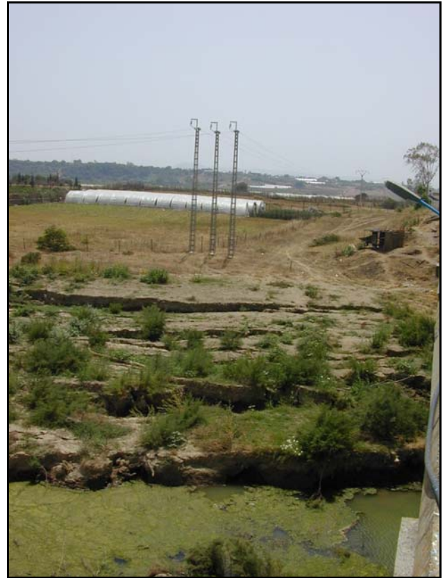
Fig. 12. Liquefaction-induced lateral spreading of the banks of Isser River
