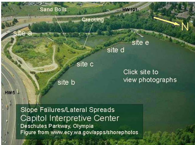
Fig. 24. Aerial oblique images are valuable in providing perspective and relative elevation changes that are not easily discern on vertical images. This image was pulled off the web and annotated to reflect locations where site damage was documented by the Berkeley reconnaissance team (from Bray, et al, 2001).
