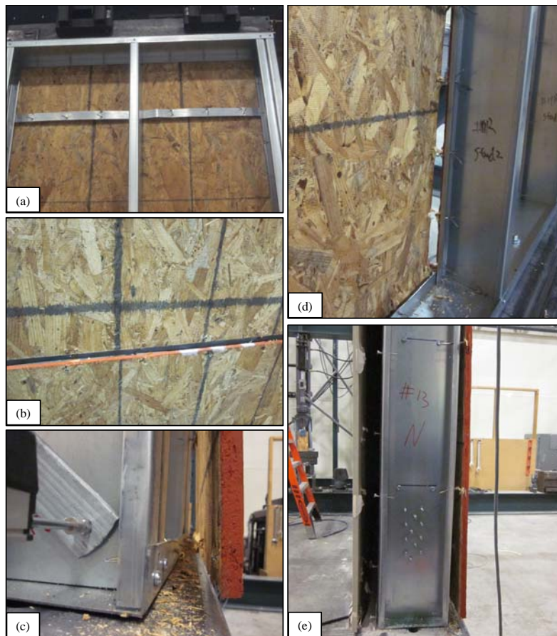
Figure 6 Detailed shear wall response (a) back of test 4, demonstrating fastener pull-through (PT) along the horizontal seam, (b) front of test 2 depicting the resulting separation of sheathing from seam as a result of PT, (c) separation of OSB from bottom of wall track in test 13, (d) Fastener PT and tear-out (TO) against sheathing along field stud in test 11, and (e) north chord stud in test 13, demonstrating fastener PT in the OSB and a combination of PT and bearing (B) in the gypsum.
