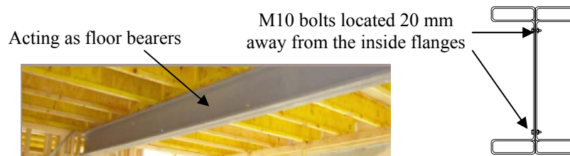
Figure 2: Back to back built-up LSBs (LST, 2005)
