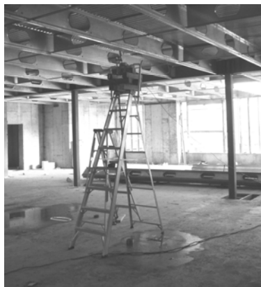
(a) Supporting Structure for Displacement Transducer
