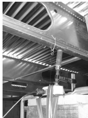
(b) Closeup of Displacement Transducer
