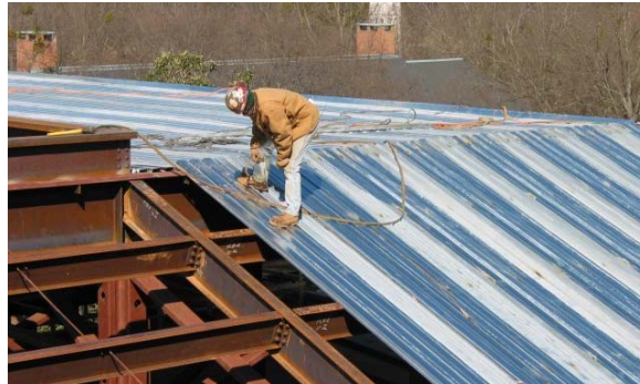
Figure 1. Arc Spot Weld Connected Roof System
