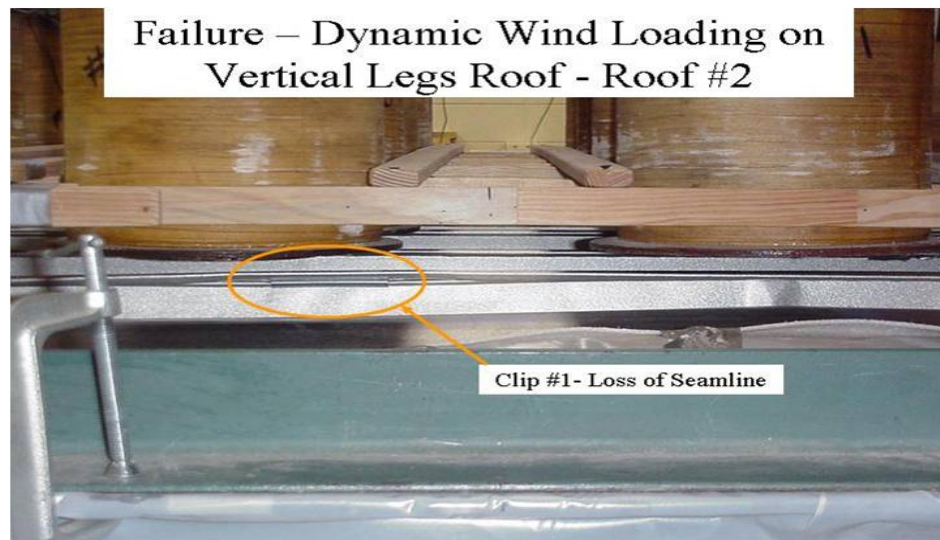
Fig 19. Failure of Clip #1 in Vertical Legs Roofs - Roof 2
