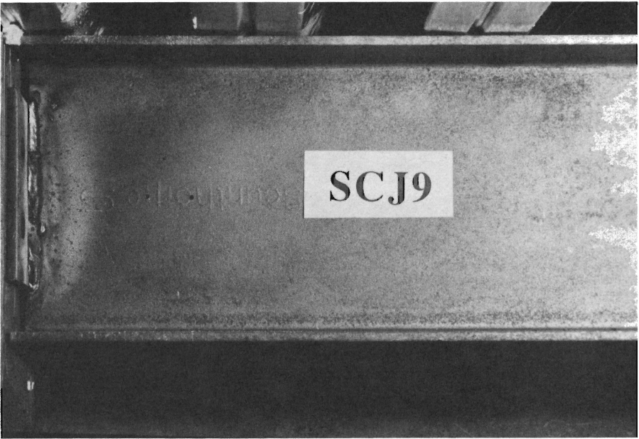
Fig.9 Eventual Failure of beam by web buckling
