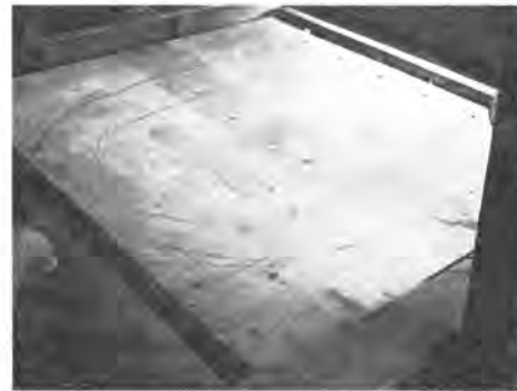
Fig. 23. Top surface of Slab 2 indicating crack pattern at termination of testing.
