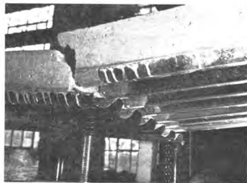
Fig. 7. Tensile steel failure of beam element.
