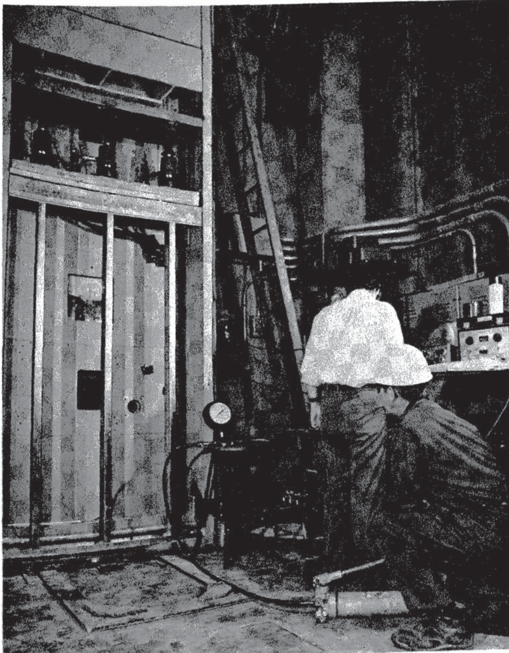
Fig. 6 Load Test Set-Up with Panel Vertical Close Up View
