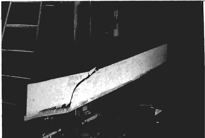
Fig. 5b: Beam No. C-4 after Failure (Shear-Bond Failure)
