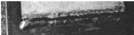
Fig. 17 Fracture of transverse fillet weld in 0.12-in sheet steel produced by Fabricator A
