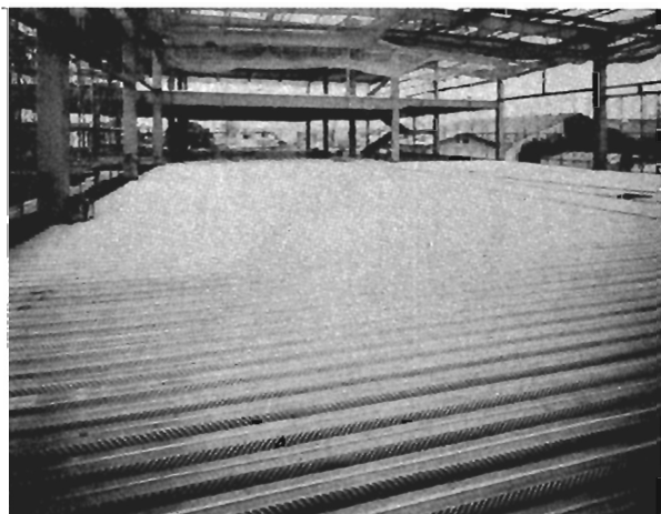
Fig. 28. Composite Floor Deck
