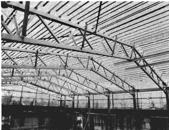
Fig. 27. Roof Trusses with Tubular Members
