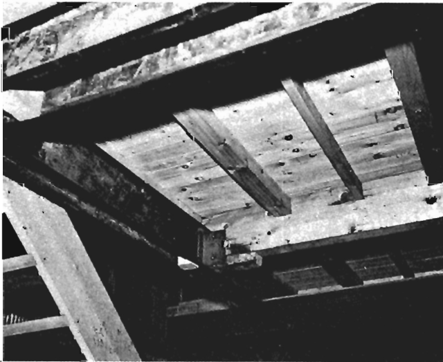
Fig. 25. Channel used in Wooden Houses
