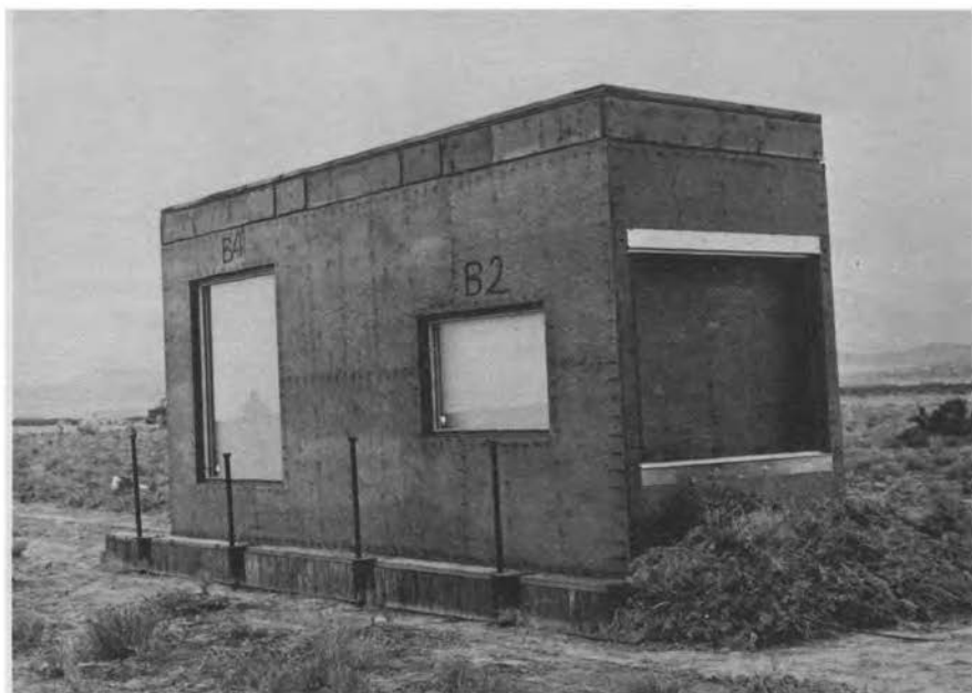
FIG. 10 - Support Structure for Explosive Testing of Cold-Formed Steel Panels (U.S Army Photograph).
