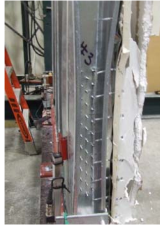
Figure 6: Screw pull out failure
