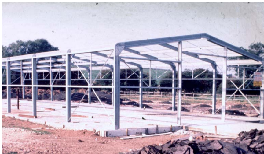
Figure 1: Cold-formed steel portal framing system
