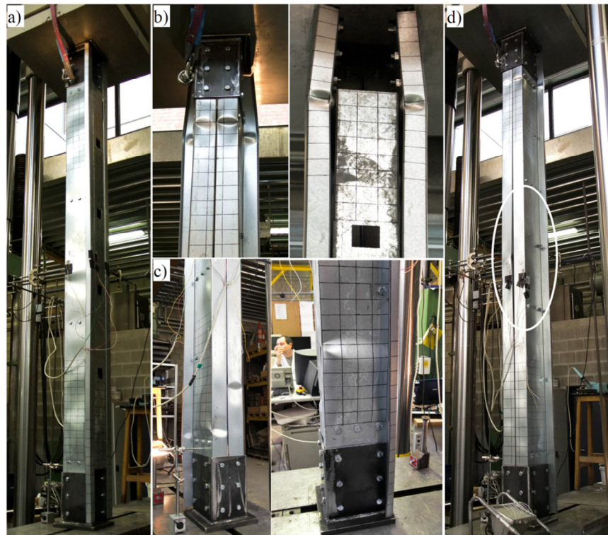
Figure 4. 2xZ200+C145 - failure mechanisms: a) local buckling; b) at top connection piece; c) at bottom connection piece; d) distortion in Z-sections.
