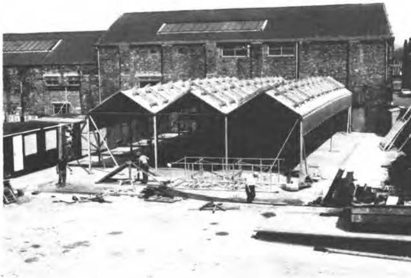
Fig 18 Full scale folded plate roof under test.
