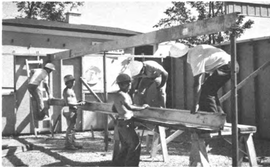
Figure 3 - Gravel Bed, Footing Channel and Basement Panels
