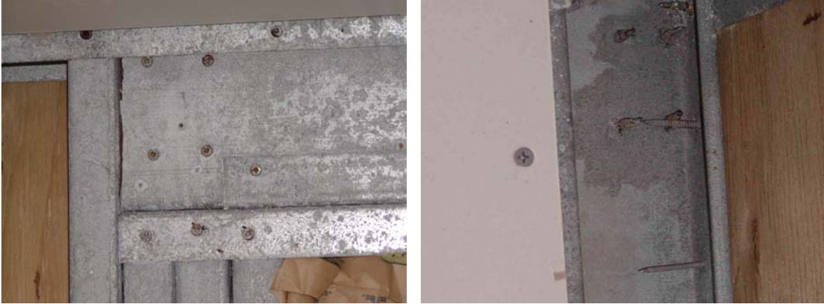
Figure 7.22: Wall framing with plywood sheathing, MCBH Coastal after 16 months.
