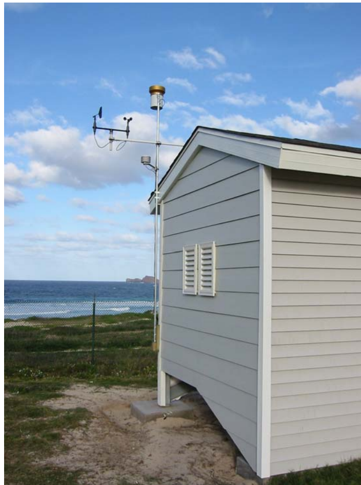
Figure 2.7: MCBH Coastal, looking NE, towards the coastline
