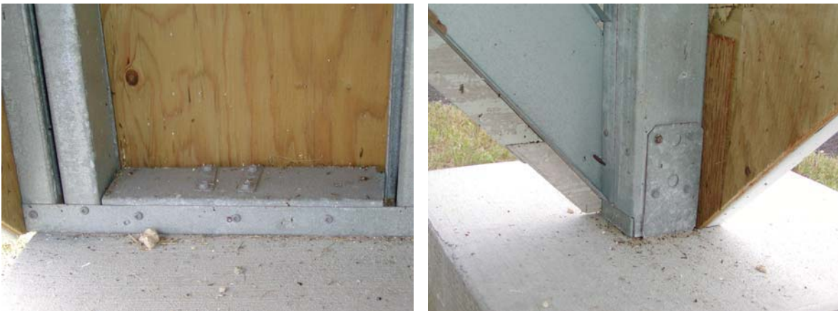
Figure 7.11: Crawl space cripple wall and post at MCBH Inland after 16 months exposure.
