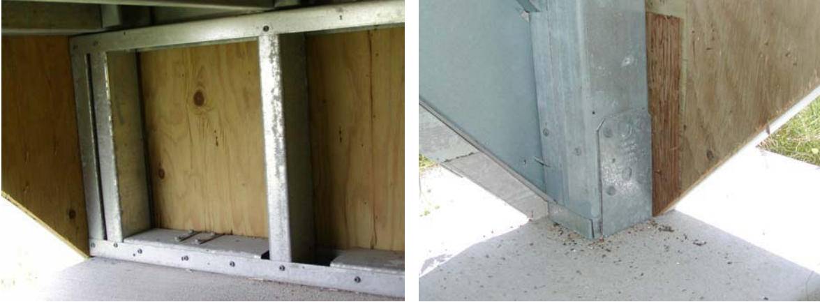
Figure 7.10: Crawl space cripple wall and post at MCBH Inland after 5 months exposure.
