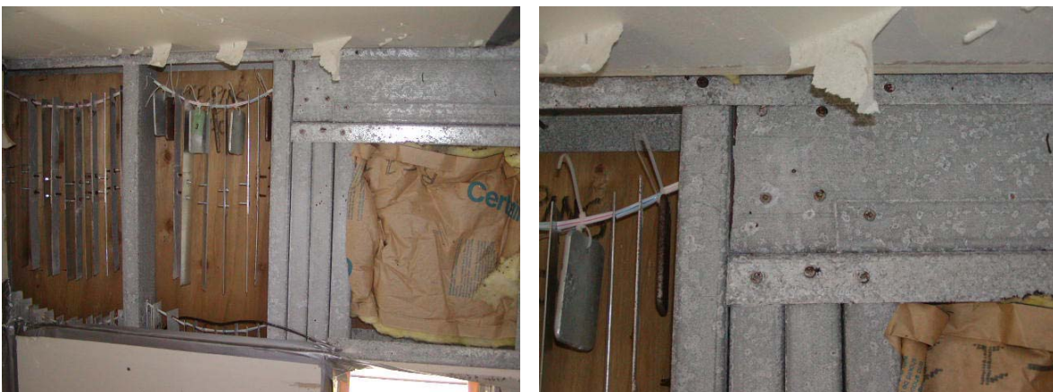
Figure 7.24: Wall framing with plywood sheathing, MCBH Coastal after 28 months.
