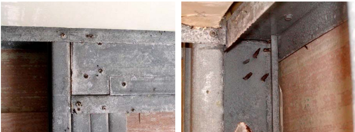
Figure 7.20: Wall framing with lap siding without vapor barrier, MCBH Coastal after 21 months.
