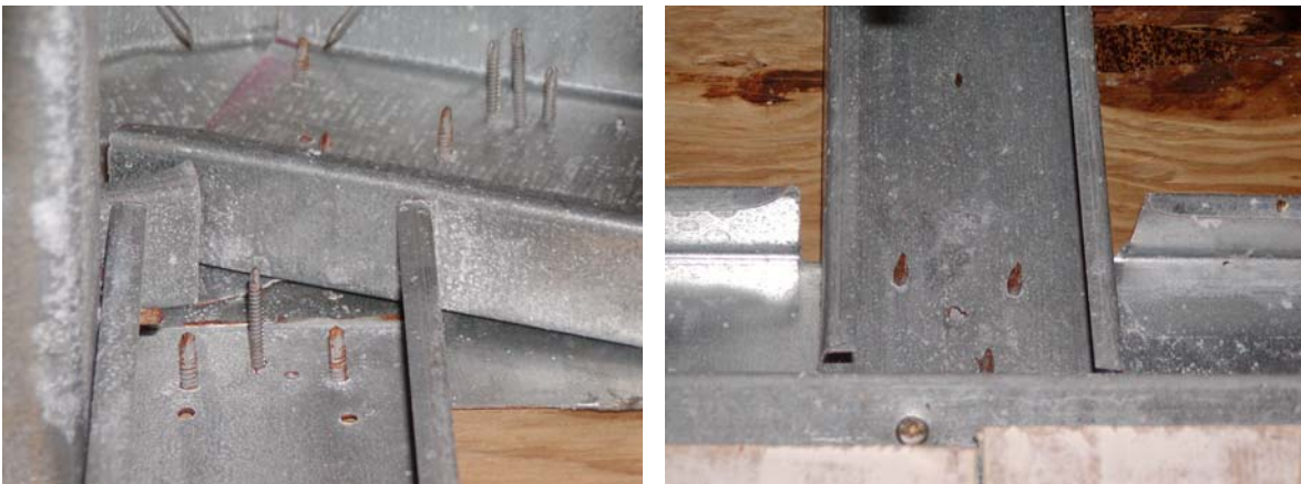
Figure 7.2: Attic framing at Iroquois Coastal site after 20 months exposure.
