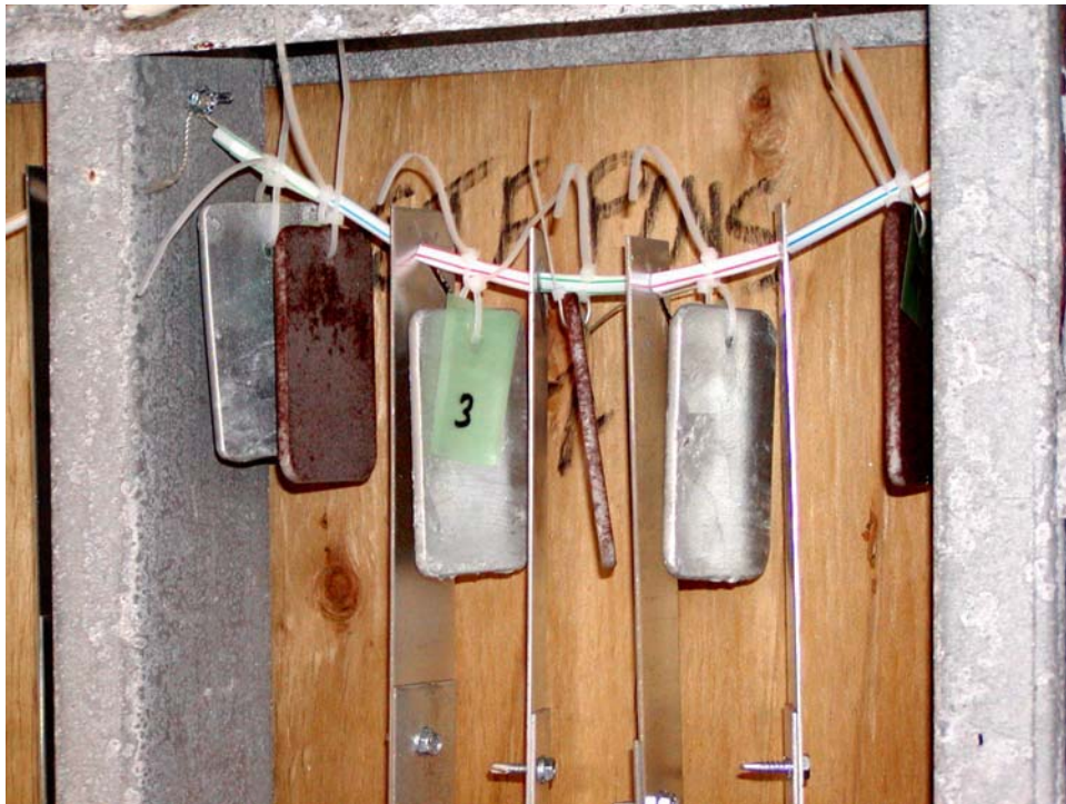
Figure 5.11: Steel and zinc coupons along with connection specimens in wall cavity.
