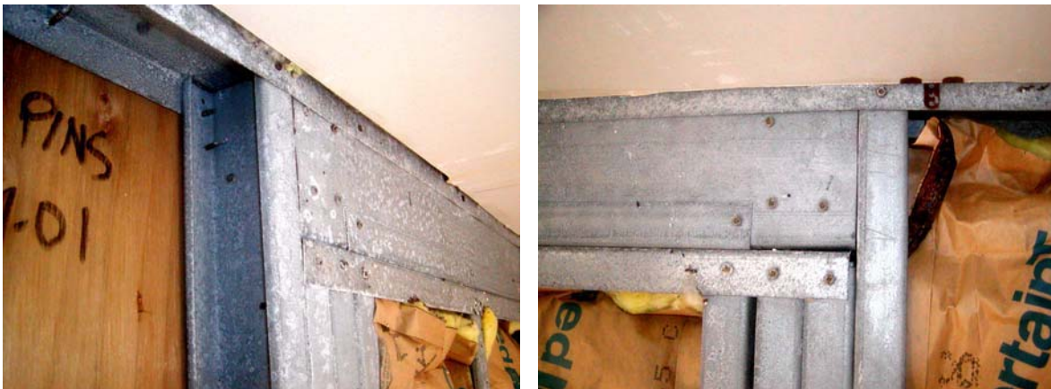
Figure 7.23: Wall framing with plywood sheathing, MCBH Coastal after 21 months.
