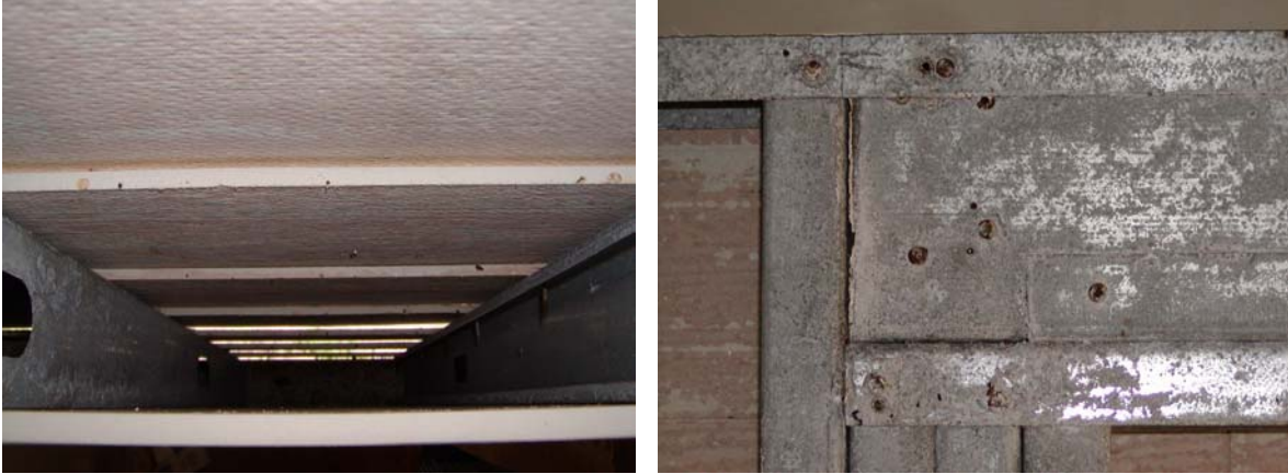
Figure 7.19: Wall framing with lap siding without vapor barrier, MCBH Coastal after 16 months.
