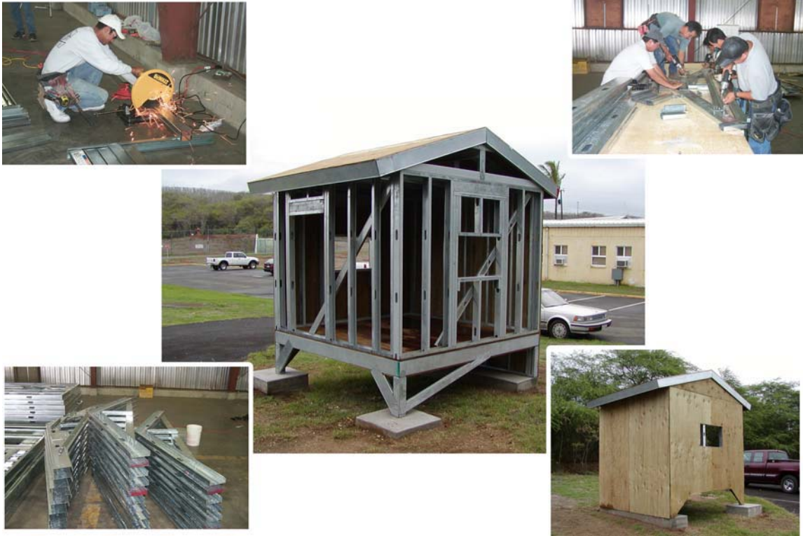
Figure 2.16: Field Enclosure at Various Stages of Construction
