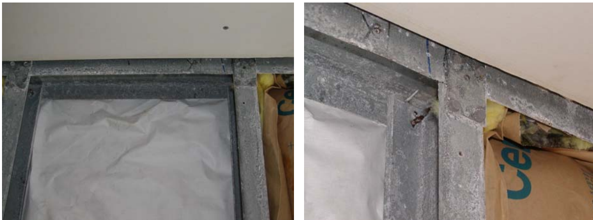
Figure 7.16: Wall framing with lap siding and vapor barrier, MCBH Coastal after 16 months.
